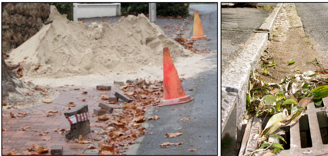
Figure 4.9: Images of uncovered sand pile and wash-off into the stormwater system. Photos taken by Elizabeth Ward.
