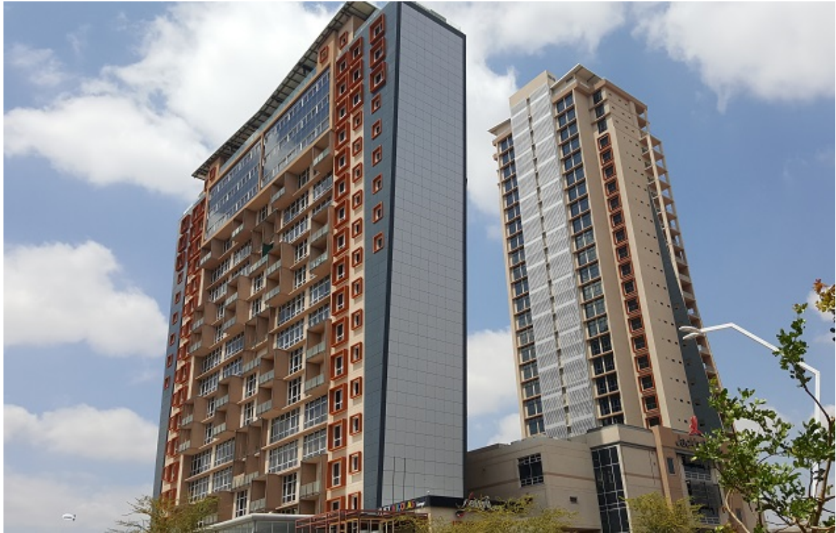
The iTowers that now mark Gaborone's new central business district. Image source: https://www.kille.bw/index.php/itowers-development-in-cbd
