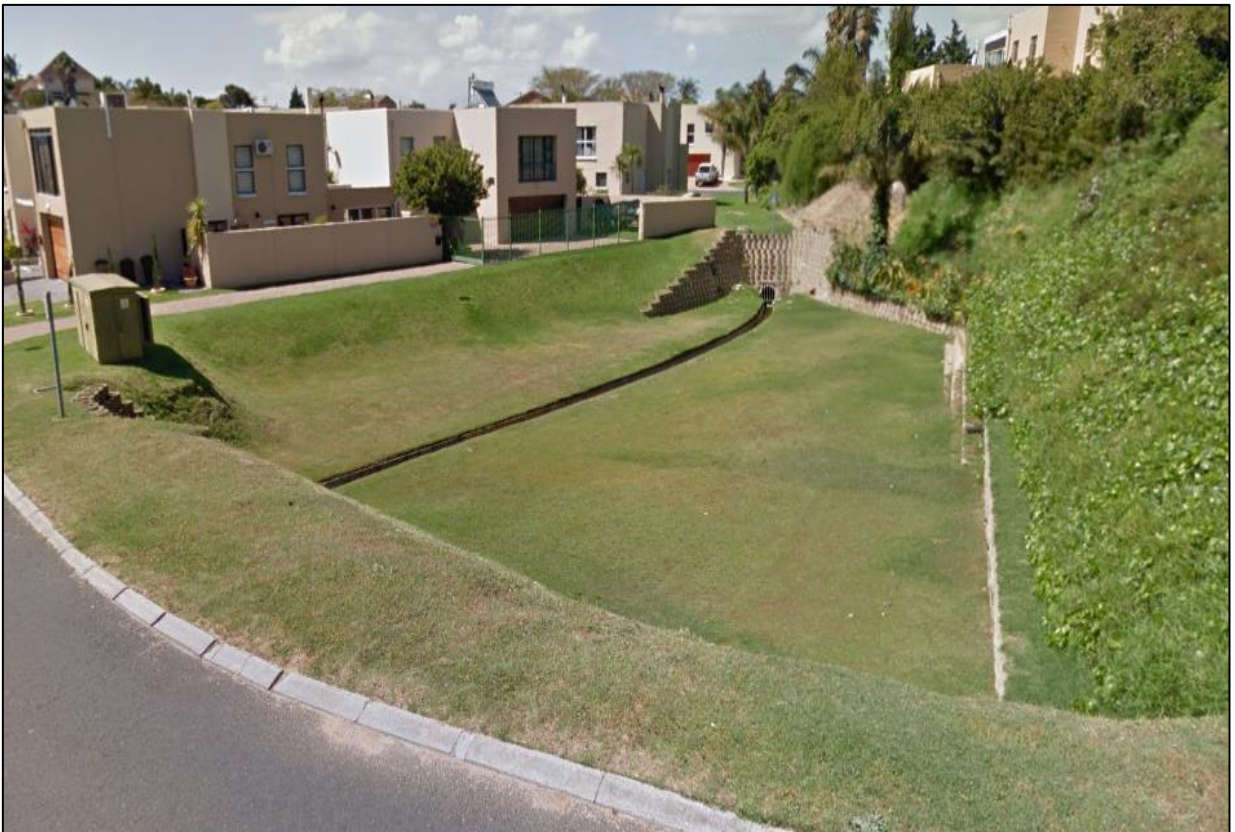
Figure 2-2: An example of a detention pond (Google Earth, 2013)
