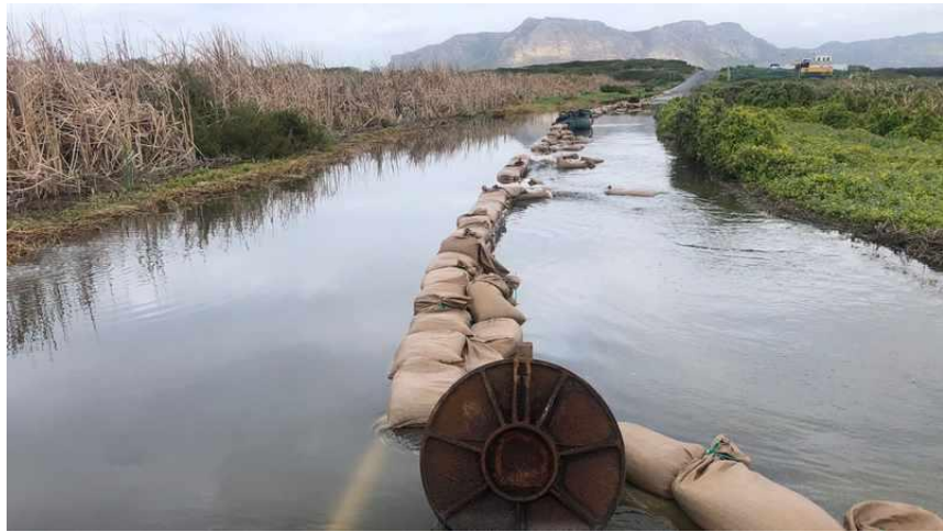
Image 5.3: Sandbags meant to contain the flow of the sewage spill. There is an open manhole caused by the sewage spill. (Source: Independent Online, 2021).
