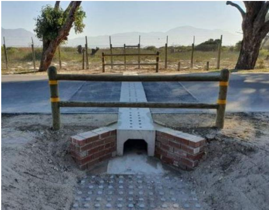
Image 6.1: Underpass tunnels built to guide toads as they migrate towards the vlei. (Source: Facebook/FOZR Facebook page).
