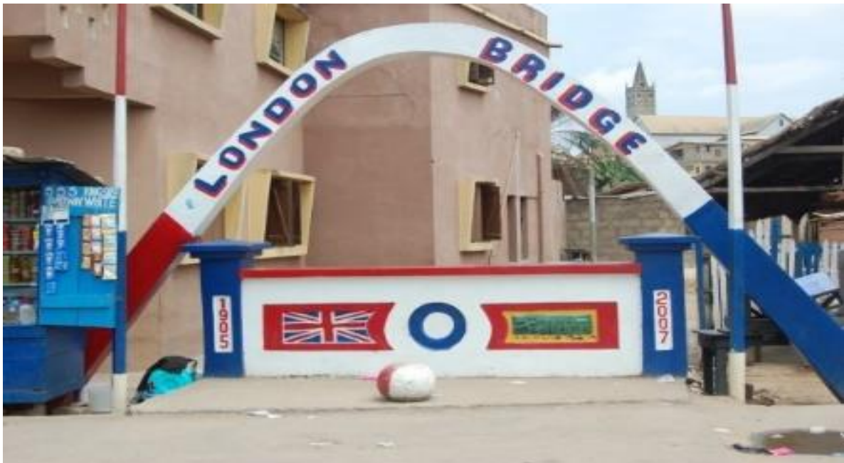
London Bridge in the centre of Cape Coast (Rashid Yakubu, 2014).
