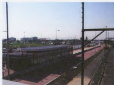
BRT route and station under construction
