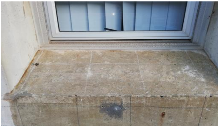
Figure 26: Location 5 (Neville Alexander building)
