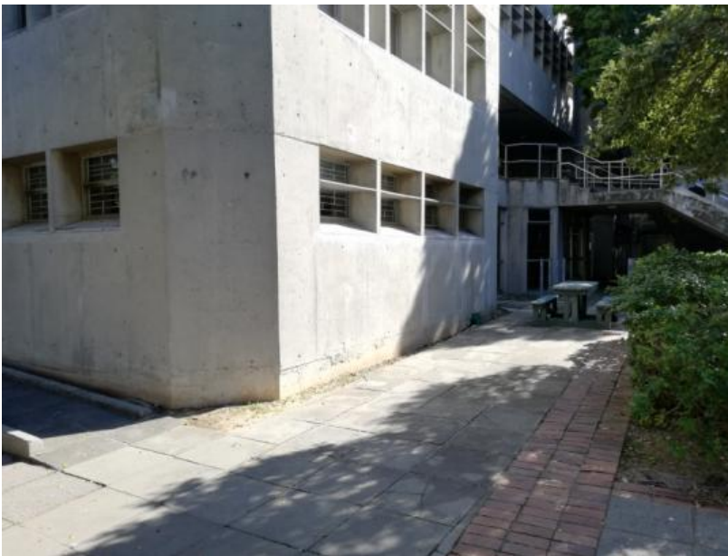
Figure 82: Location for the cover depth assessment on the ground floor of the east side of the Neville Alexander building zoomed out
