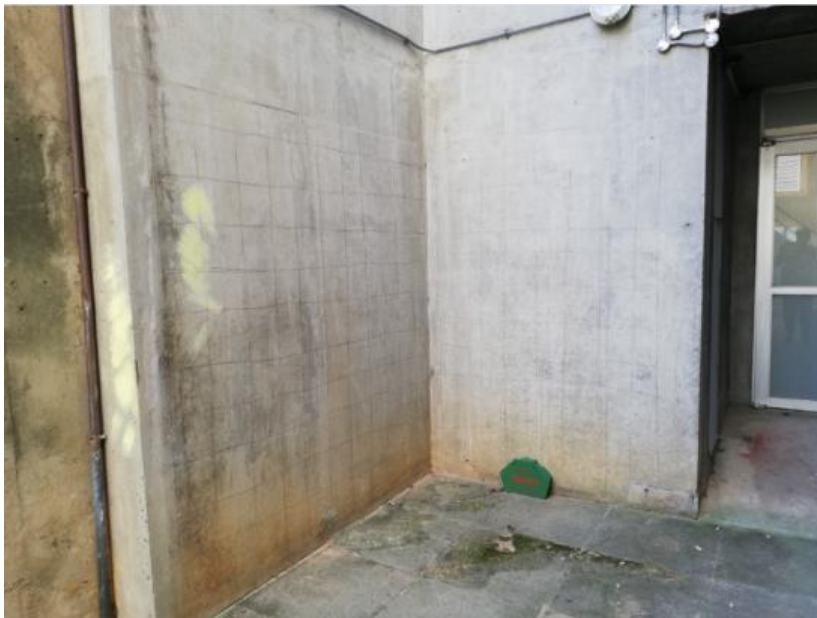
Figure 37: Large location for the cover depth assessment on the ground floor of the west side of the Neville Alexander building
