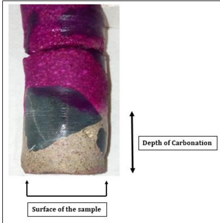
Figure 9: Indicator colour change on a carbonated concrete sample
