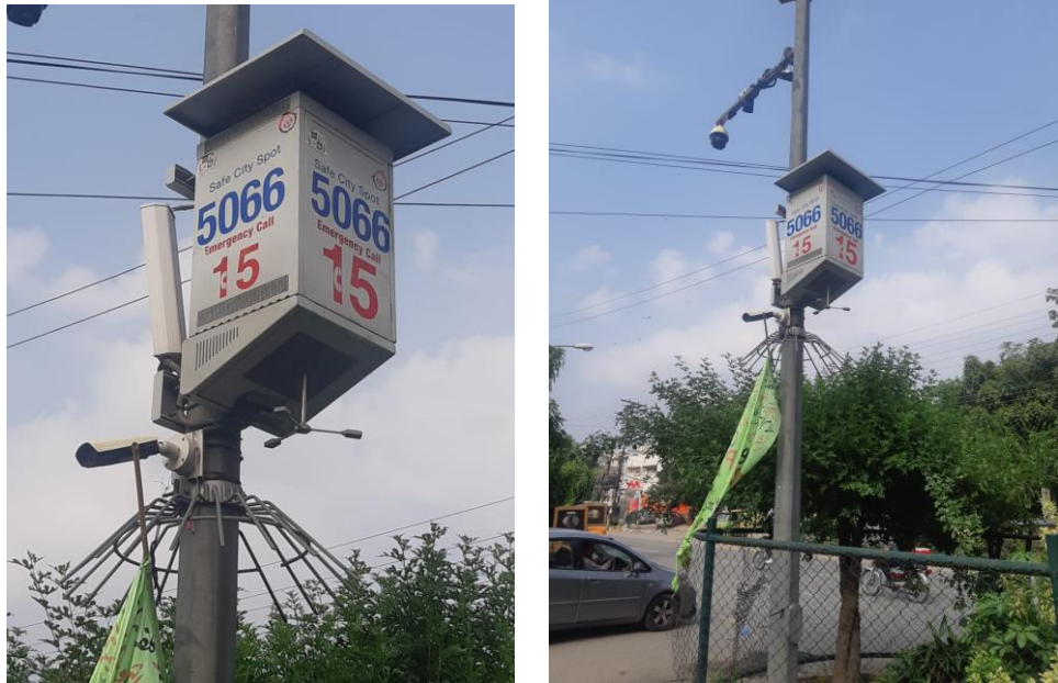
Figure 33 CCTV Cameras PSCA Lahore
