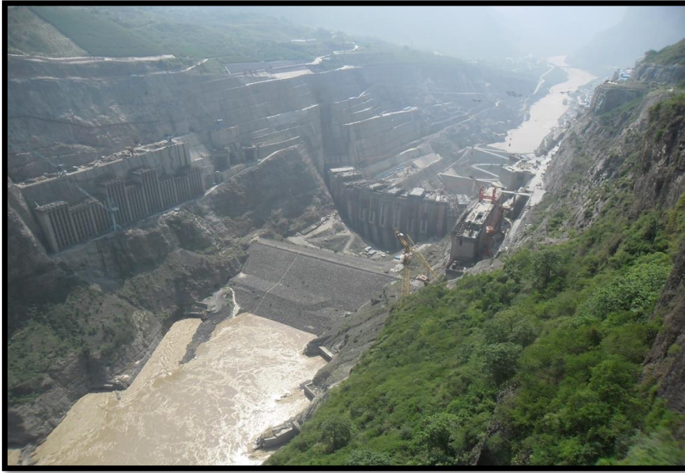
Figure 2.3: Xiluodu Dam ("Xiluodu Dam, Jinsha River, China". Water Technology, 2014).
