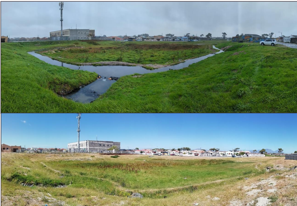
Figure 4-4: The study site during wet (top) and dry (bottom) conditions. In both pictures the forebay area in front of the southern inlet is visible.
