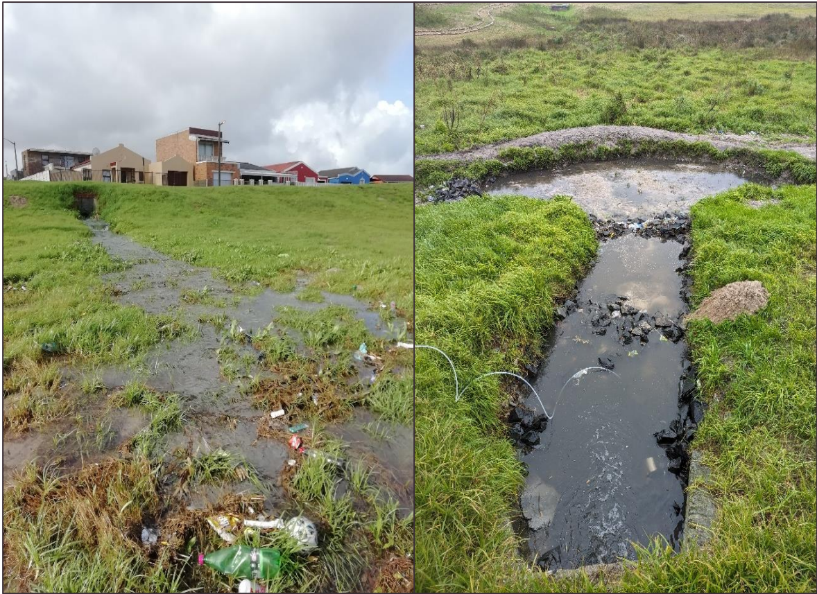
Figure 4-7: Stormwater inlet showing overland flow before swale construction (left) and stormwater containment by swale with stormwater sampling tube (right).
