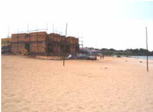
(c) Accommodation rooms being constructed right on a sand beach
