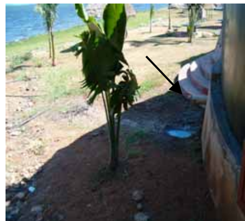
(f) Wastewater flows to the lake through a Kitchen drain pipe
