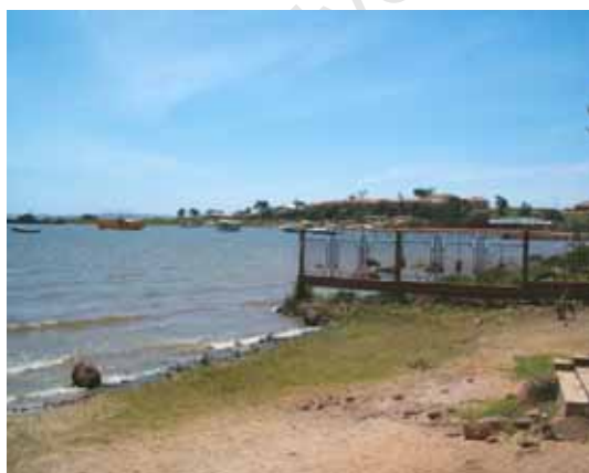
(e) Sites fence off their premises right into the lake
