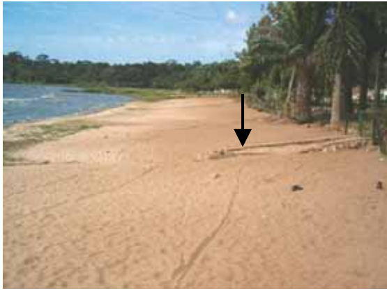
(a) Storm water drain provision at a beach
