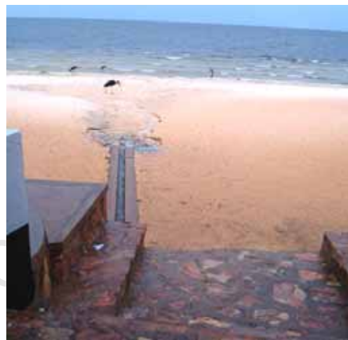
(d) Storm water flowing into the lake
