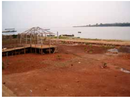
(b) Infilling and landscaping of part of the lakeshore originally under water
