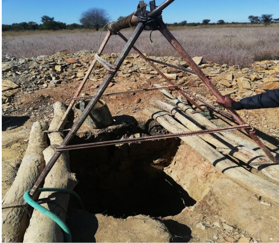
Figure 4.16: Shaft hoist with loading bucket attached (authors own)
