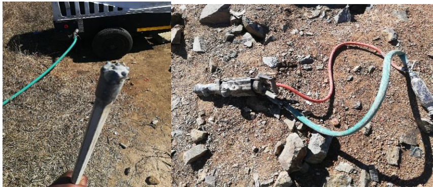
Figure 4.15: Drilling Equipment (authors own)
