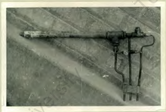
Laboratory kiln, burner-pipe, and coal-bin. (See page 138.)
