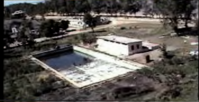
FIG 20 2009,View of the front of the swimming pool area of the Grand Hotel Beira
