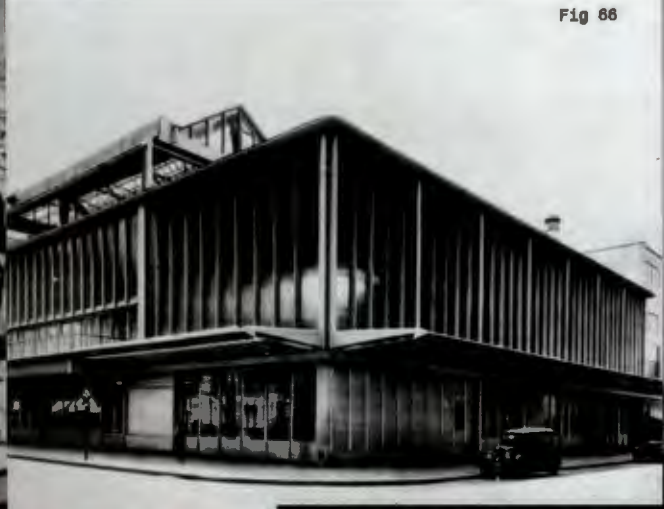
MAISON DU PEUPLE by JEAN PROUVE It was one of the earliest examples of a unitized curtain wall system that radically altered the way future buildings would be built.
