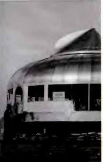
MAISON DU PEUPLE by JEAN PROUVE It was one of the earliest examples of a unitized curtain wall system that radically altered the way future buildings would be built.
