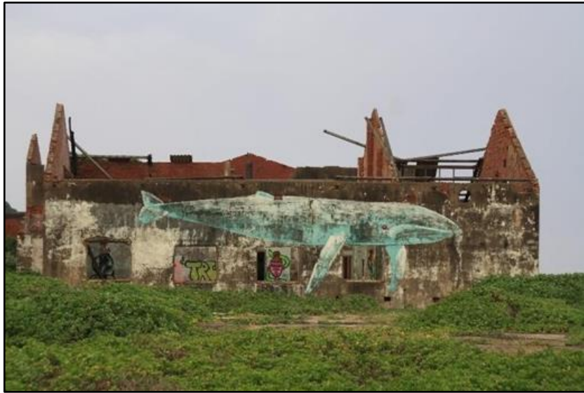
Figure 9 Delapidated building structure with graffiti, located at the Whaling Station (Liversage 2017)
