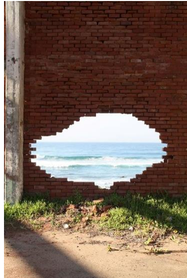
Figure 12: Hole in Whaling Station Warehouse, overlooking Durban ocean (Liversage, 2017)
