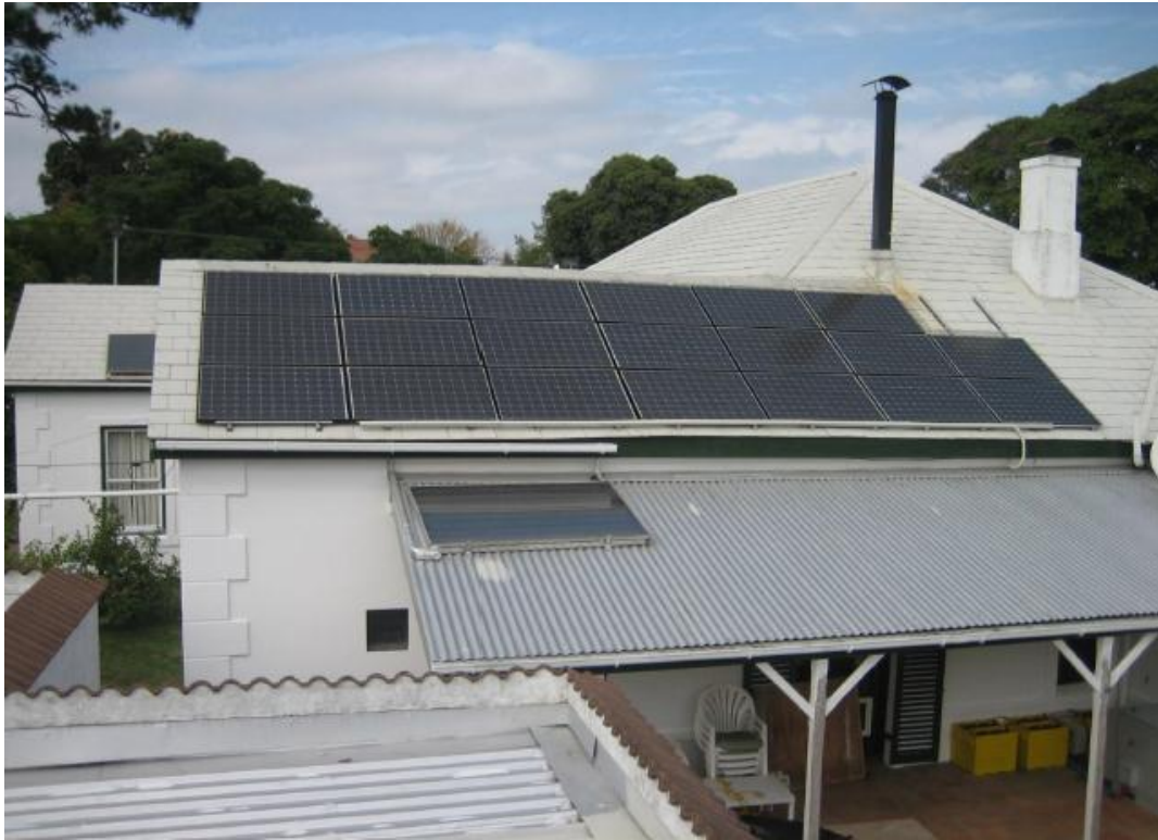
Figure 3: The 3.8kWp PV array at the home of Dr. Keen, who is partaking in the pilot project with the city of Cape Town on net metering. Taken from (Keen, 2012).
