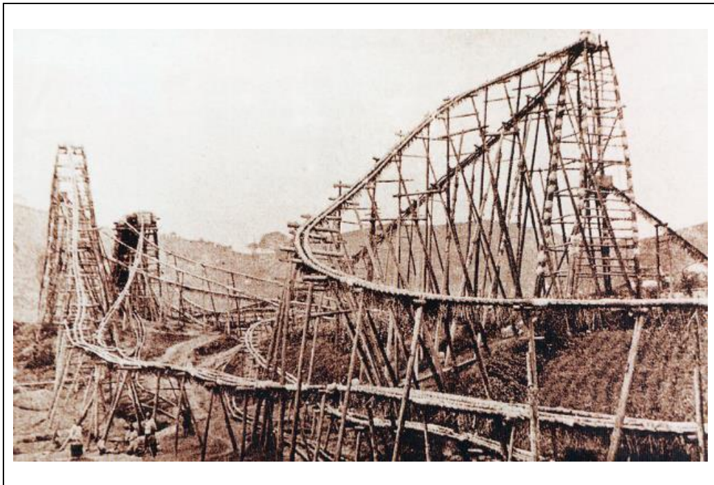
Figure 1.1 Early 20th century photo of gravity-driven bamboo pipelines used to transport brine and natural gas in China. It was reported that bamboo pipelines covering a distance of up to 95 km were in operation until the 1950s in China. Source: Kuhn (2004)
