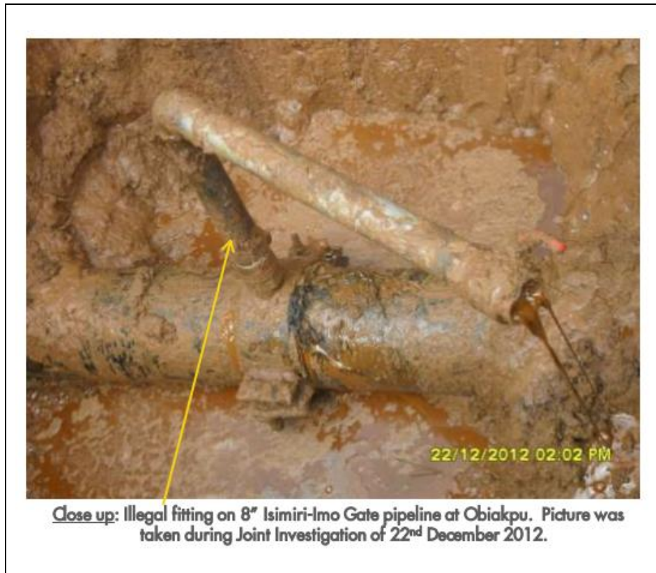
Figure 5.5 The JIV photograph of the spill source due to sabotage of the Isimiri-Imo pipeline at Obiakpu on 22th December 2012.
