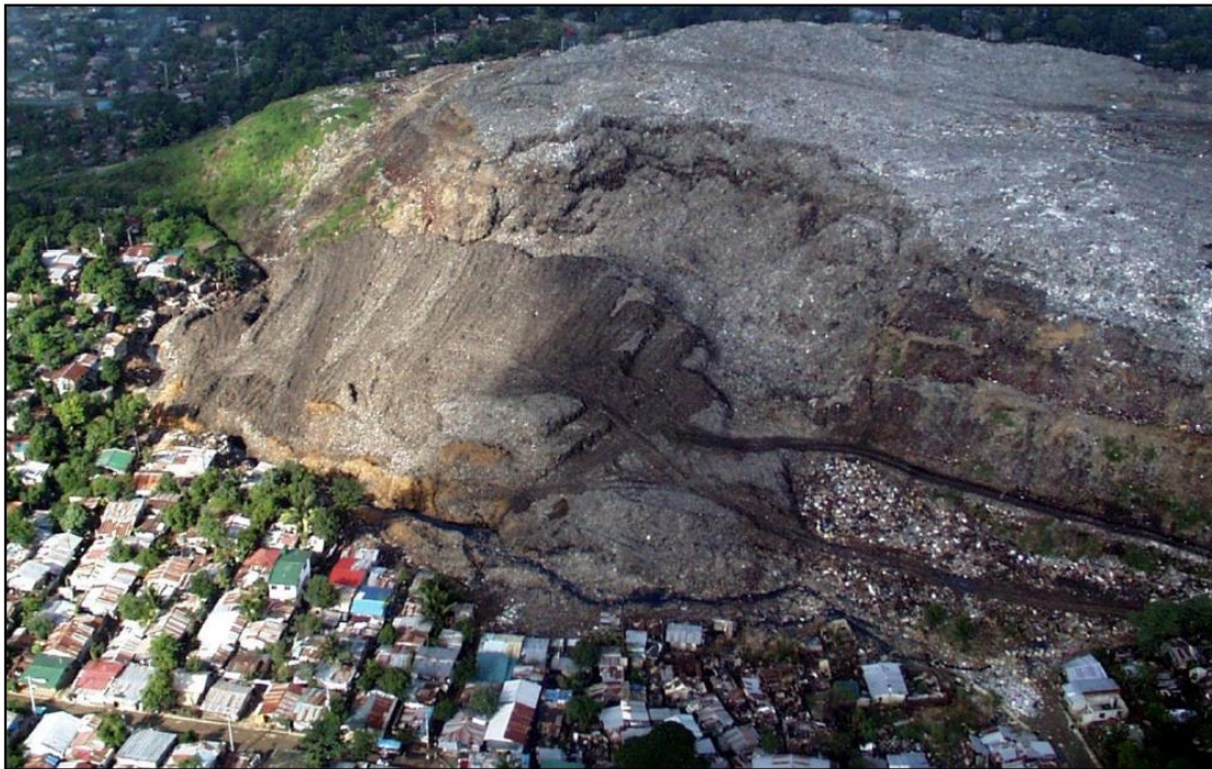
Figure 3-2: Aerial view of Payatas landfill with slope failure and homes visible in foreground (Jafari, et al., 2012)
