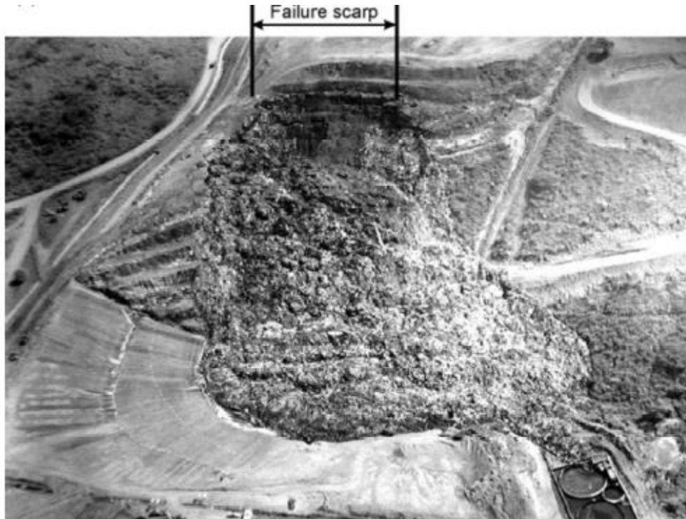
Figure I-4: Bulbul landfill failure at Durban, South Africa (Blight, 2008)
