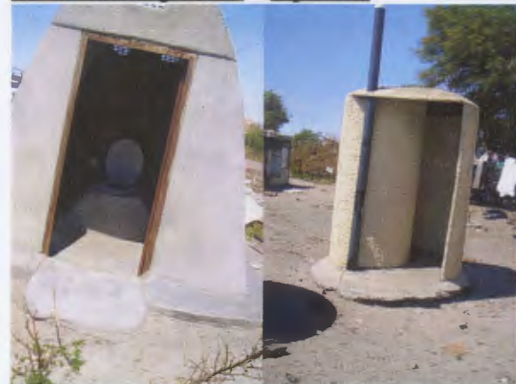
VIP toilets: Figure 28 Figure 29
