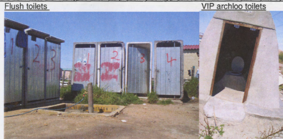
Figure 13: Photo's of the types of toilets presently being provided to Informal settlements by CCT
