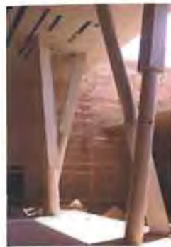
The foyer of the new Constitutional Court building, presently under construction
