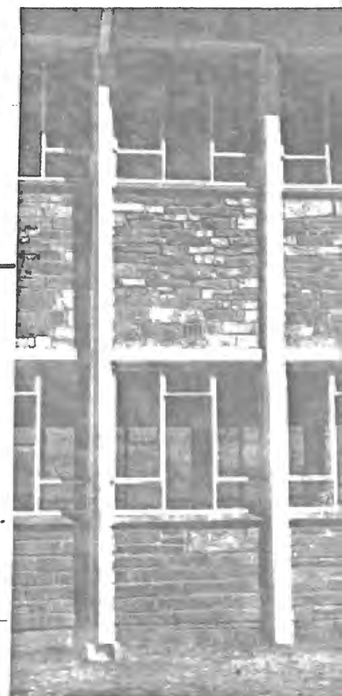
Bay detail : showing steel windows and Quithing stone panels.
