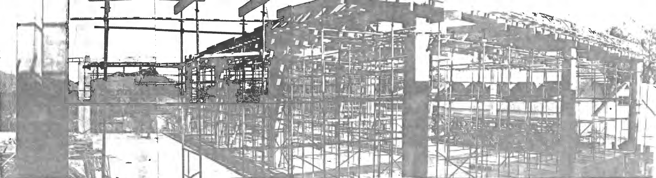
EXCAVATION ( below ), Lesotho Hilton and FORMWORK & PROPPING ( above ), Liquor Commission, Maseru
