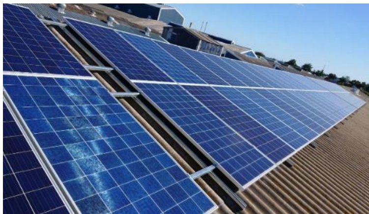
Figure 55: Mounting of the photovoltaic modules at SA Tyre Recyclers
