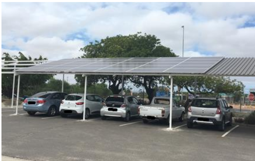
Figure 51: Completed installation of the photovoltaic system at SAREBI
