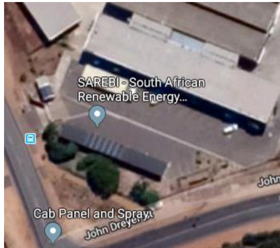
Figure 50: Aerial photo of SAREBI ground-mounted structure (Google Earth, 2019)
