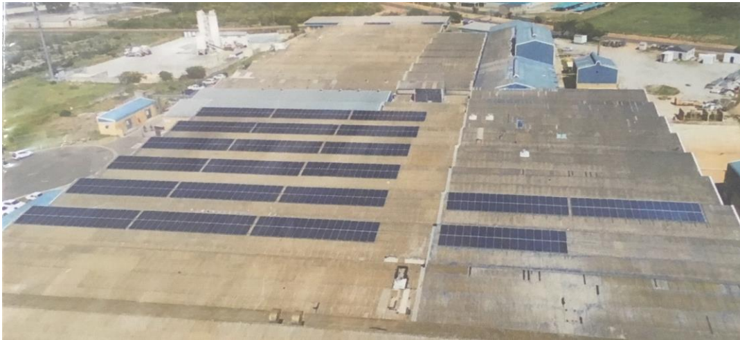
Figure 54: Drone footage of the completed photovoltaic system at SA Tyre Recyclers
