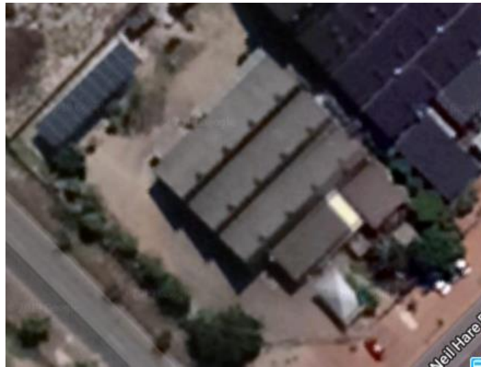
Figure 56: Aerial photo of the Stripform Packaging solar photovoltaic system (Google Earth, 2019)
