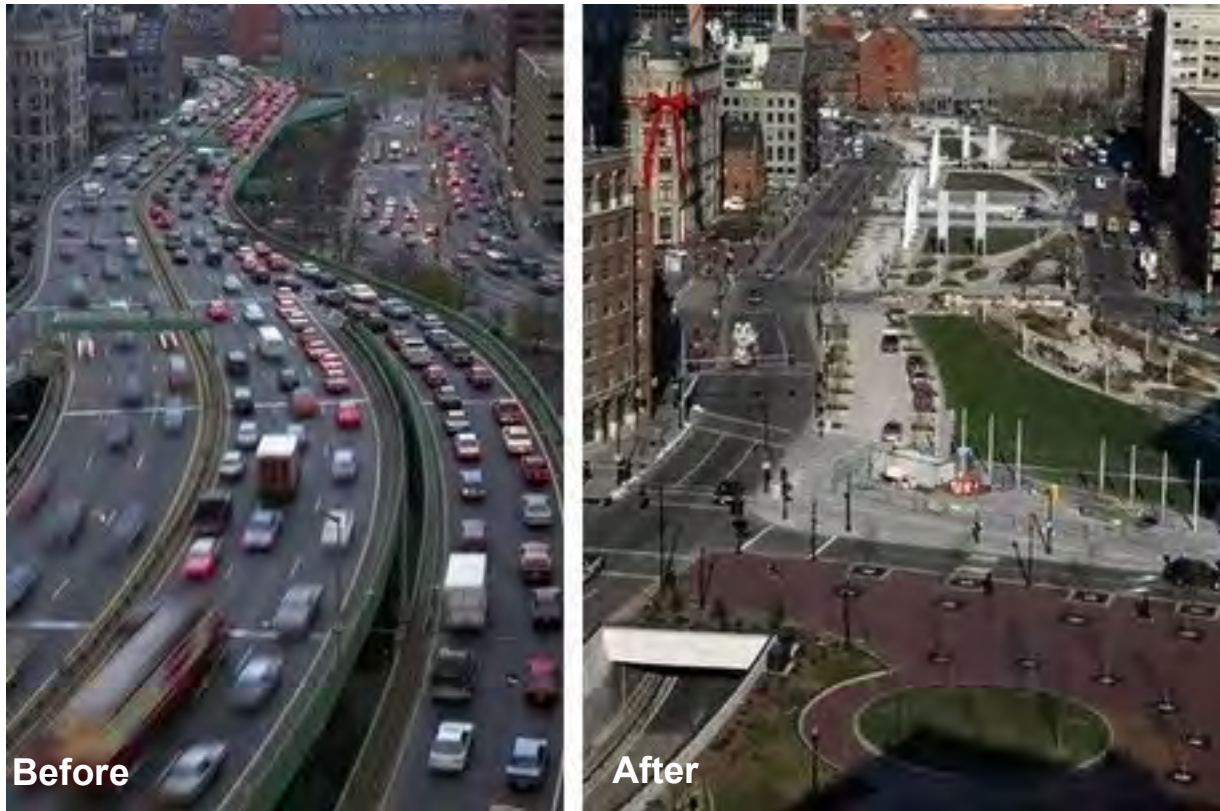
Before and After pictures of the Boston Big Dig Central Artery project showing the use of a tunnelled freeway ( www.skyscrapercity.com , 2011)
