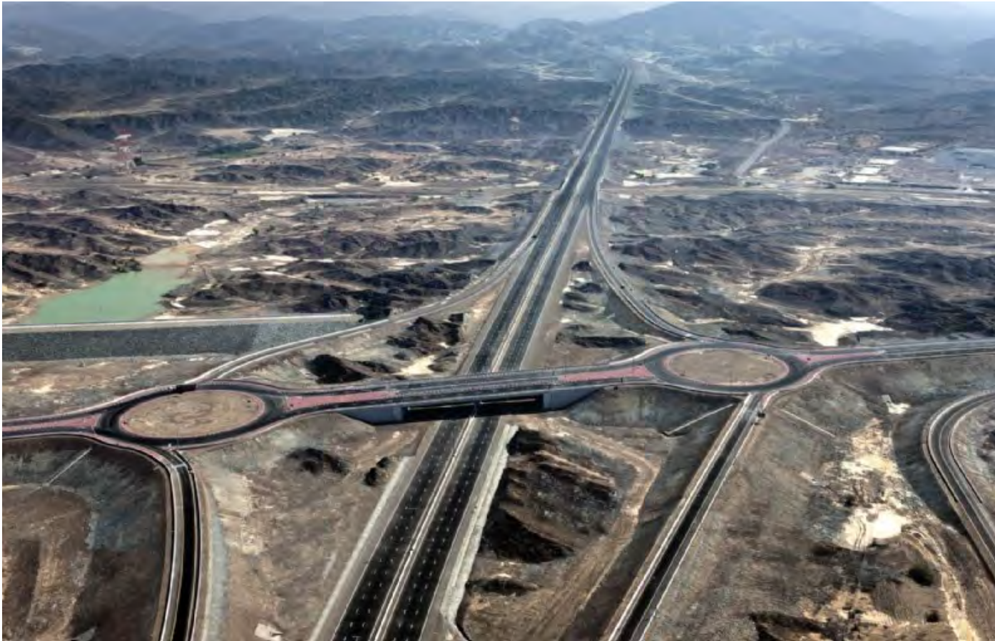
Embanked freeway structure of Dubai-Fujairah-Freeway
