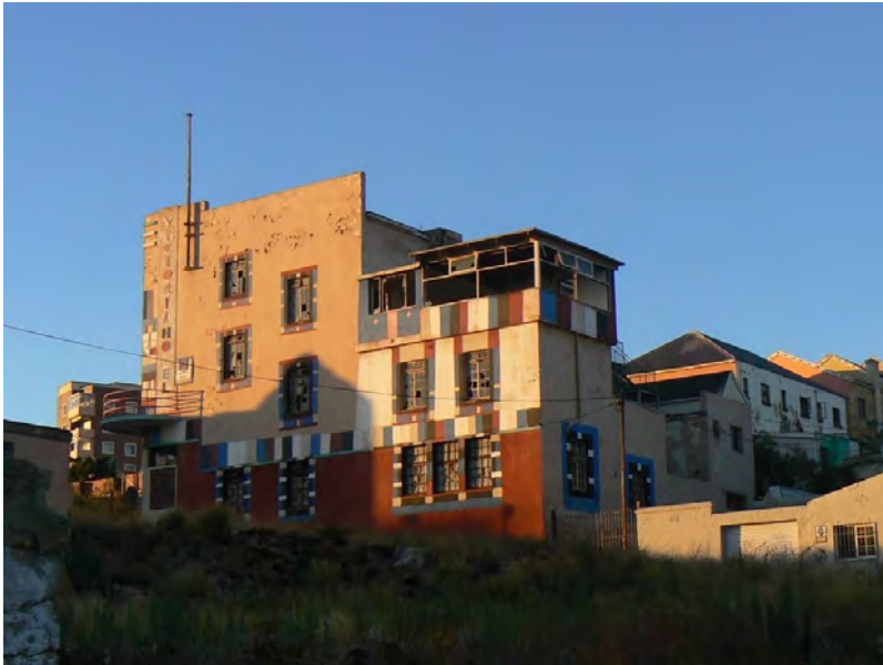
The derelict Victoria Hotel in Central ( www.portelizabethdailyphoto.com , 2009)
