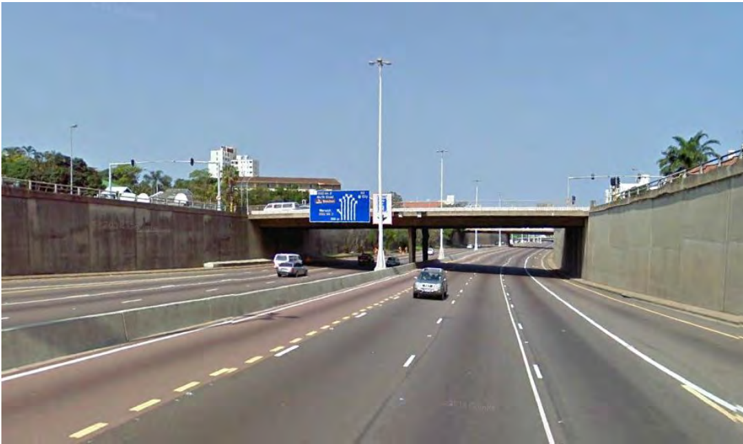
Depressed freeway in Durban moving through a city (www.googleearth.com, 2014)
