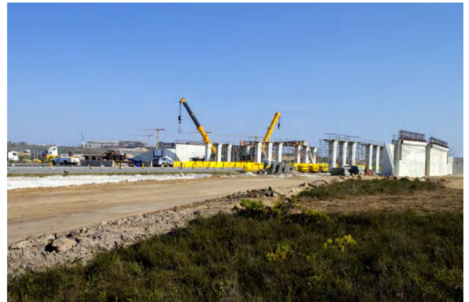
Construction of freeway infrastructure for the new Baywest mall ( www.baywestmall.co.za , 2014)
