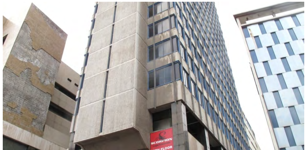
Derelict buildings in the inner city of Port Elizabeth ( www.simpleintrigue.blogspot.com , 2012)
