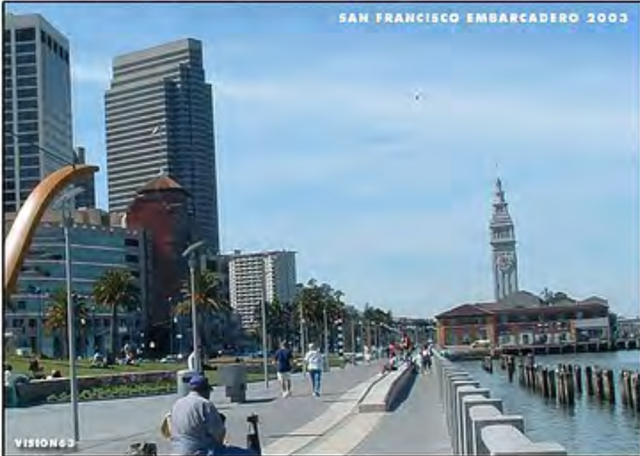
Embarcadero Freeway in San Francisco before and after demolition (www.prologspier1.com, 2014)
