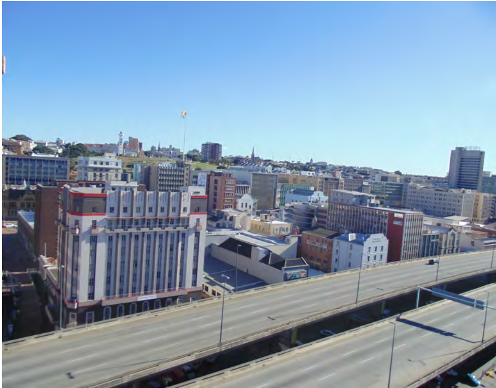
Elevated Side-by-side freeway in Port Elizabeth (author, 2014)
