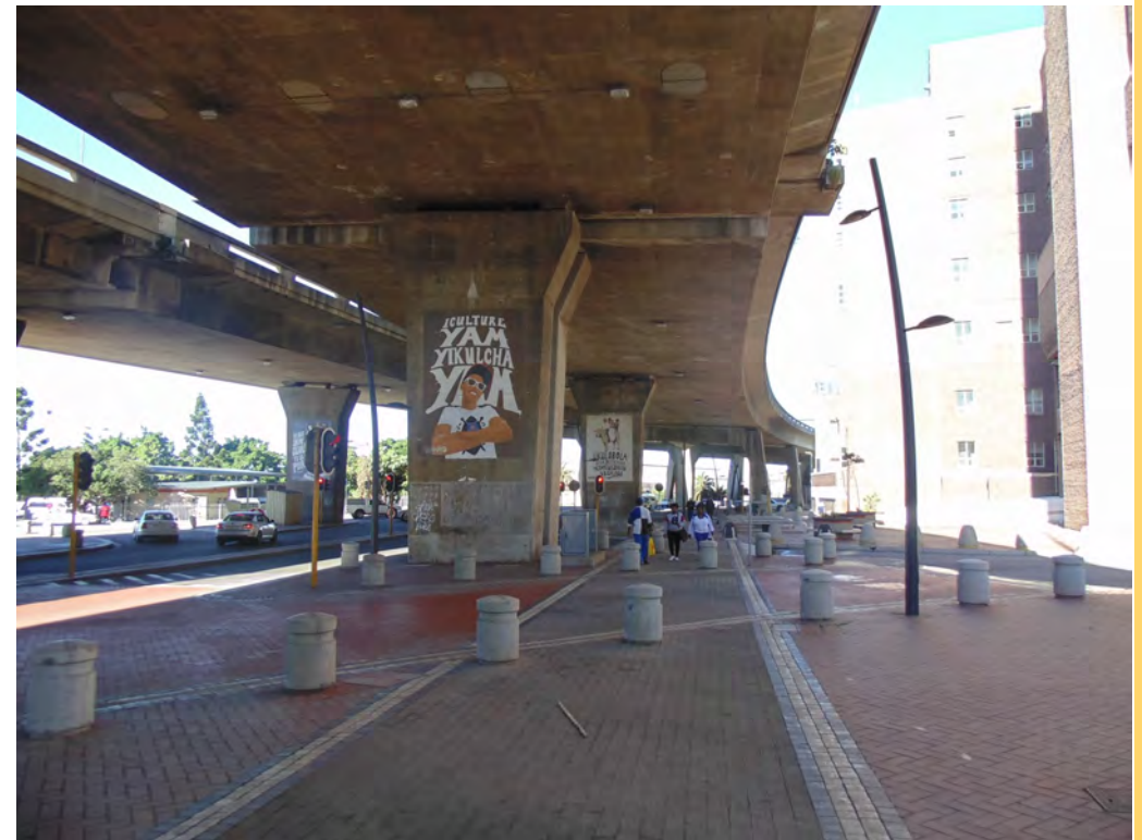
Underside of elevated freeway in Port Elizabeth (author, 2014)
