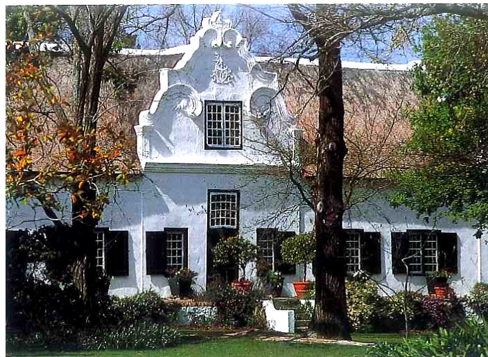
Figure 11: West Gable of the Ida's Valley Homestead (Simons 2000:118)
