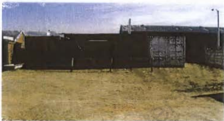
CHPA old treatment area.
