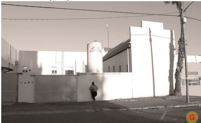
Figure 40.2 : Back of the Hospital building Park Avenue Source: Author(2022)
