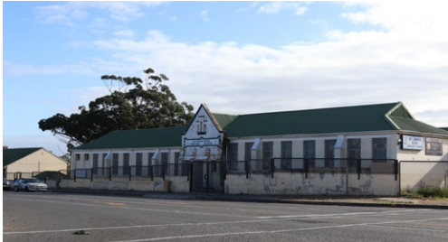
Figure 172: St Johns Road Primary School. Source: Author (2022)
