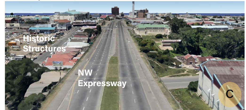
Figure 38.6: Current perspective of the North West Expressway Source: Google
