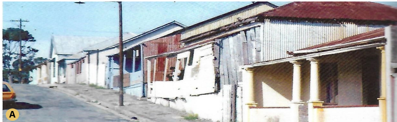
Figure 32.2.2: Perspective of St Johns Road houses build the street
