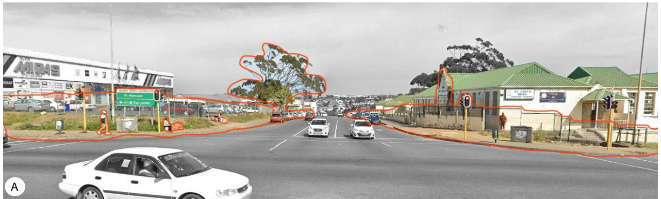
Figure 42.4 : ST JOHNS ROAD & NORTH WEST EXPRESSWAY INTERSECTION Source: Author(2022)
