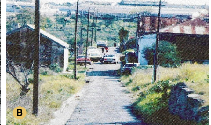
Figure 32.1.2: Ryans Lane during demolition. Source: Rangasamy (2018)
