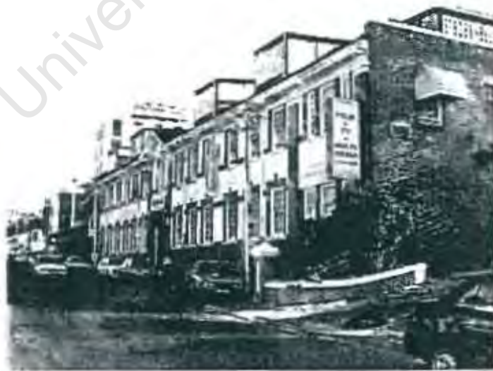
Fig. B3/6 Boston College along Klout Street (Building 5 or administration building).
