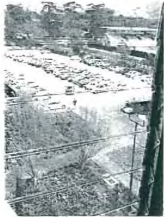
Fig. B4/6: View across upper deck of new parking (from top of Manendahl Sewer)
