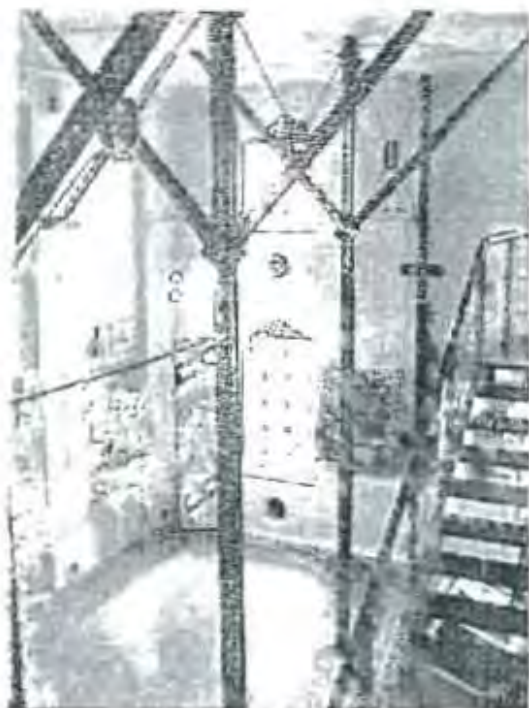
Fig. B4/20: highlighting of the original structure
