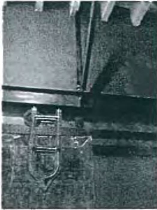
Fig. B3/27 Detail of an old fire door (reused as part of a wall)
