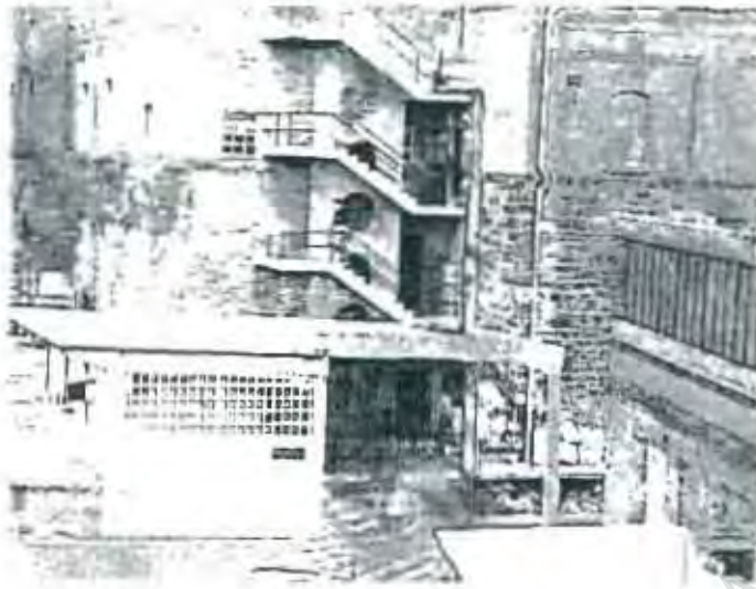
Fig. B2/10: The new staircase, also used as fire escape
