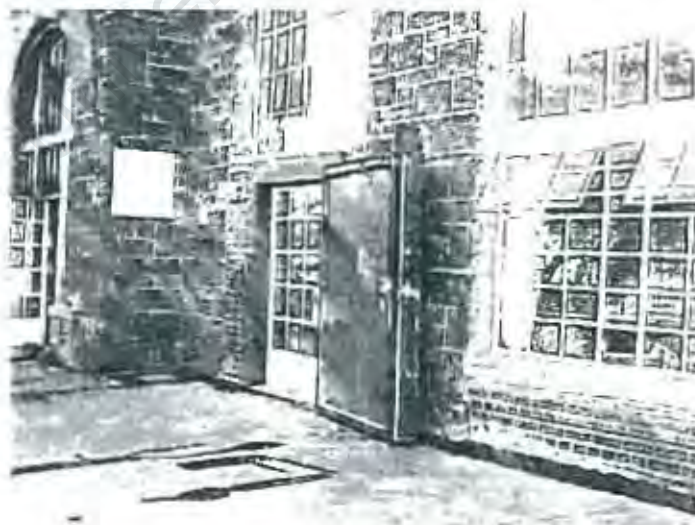
Fig. B3/23 Remaining bridge door in front façade
