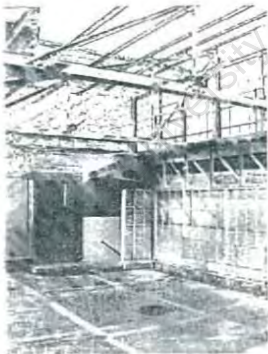
Fig. B2.8 The space that was intended to be part of a pub
