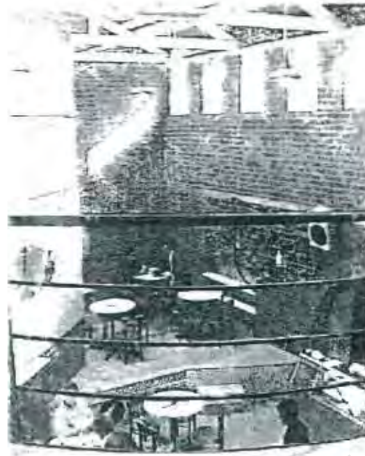
Fig. B3/15 Interior of baler house, view from new mezzanine floor
