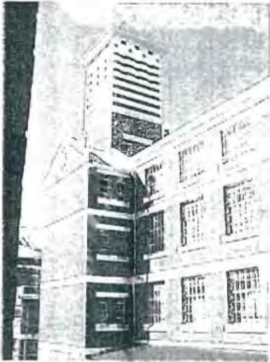
Fig. B3/19: Part of Building 2 with water tower at the back, showing the red face-brick with white plastered bands
