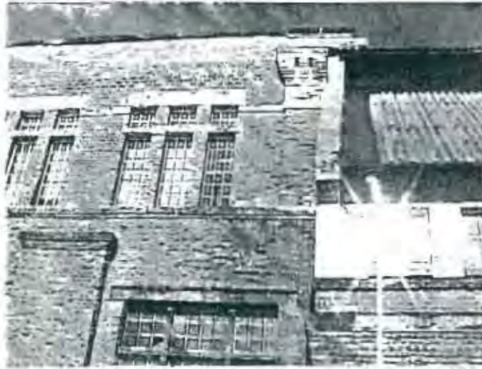
Fig. B2/22 View of original brewery building (left) and addition that was retained (right)
