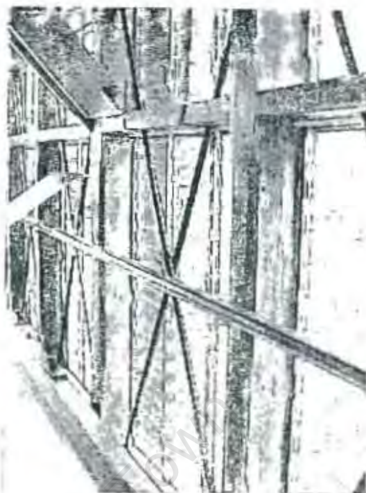
Fig. B4/21: View of 'cleaned up' original structure on top level of Mariendahl Brewery
