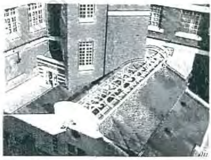
Fig. B3/14 The boiler house
