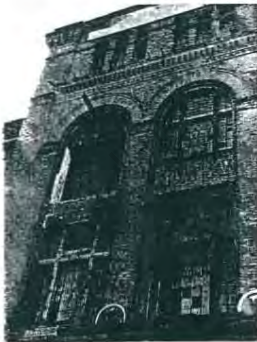
Fig. B2/17: The rundown state of the building before the 1984 conversion (detail of front façade)
