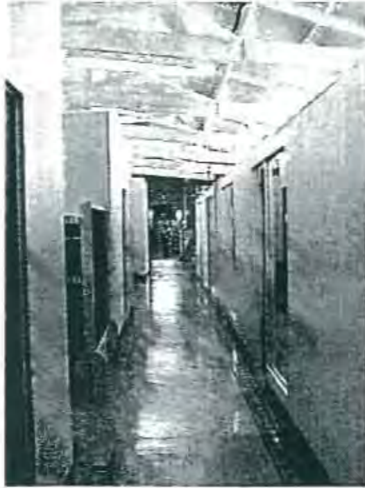
Fig. B3/17 Internal subdivisions in one of the open-plan spaces, original structure partly visible
