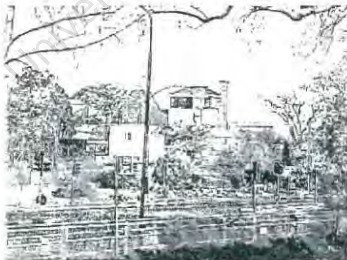
Fig. B4/34 View of site from Main Road
