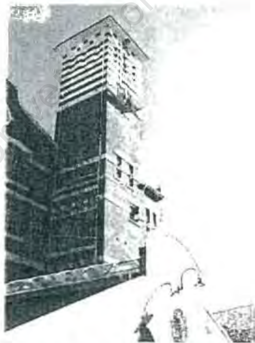
Fig. B3/4 The water tower
