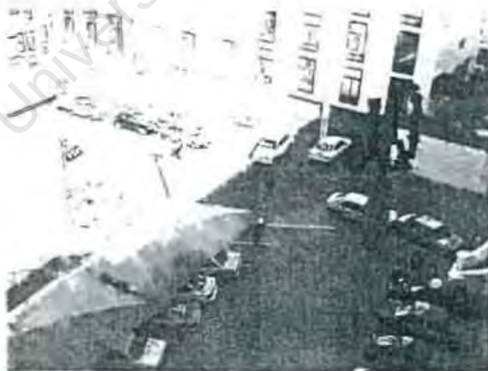
Fig. H3/12: View of the new parking bays in front of Building 1 and Building 2 - on the location of the demolished Bernmore house (after the conversion)
