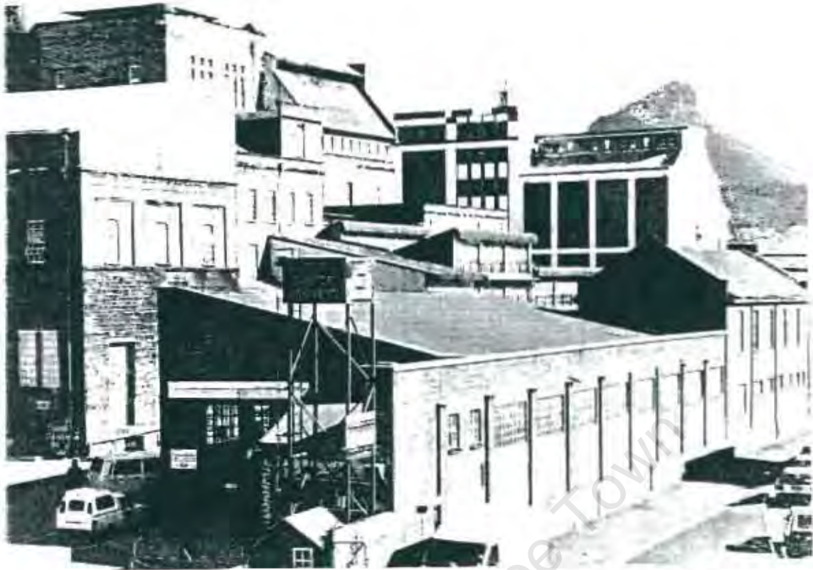
Fig. B2/16: View of entrance to the stables in front and canopy attached at the right
