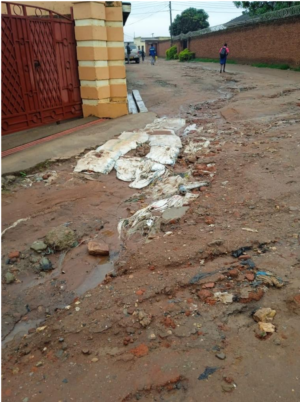
Figure 11: Use of Sand Bags to prevent soil erosion on roads (Source: Researcher)
