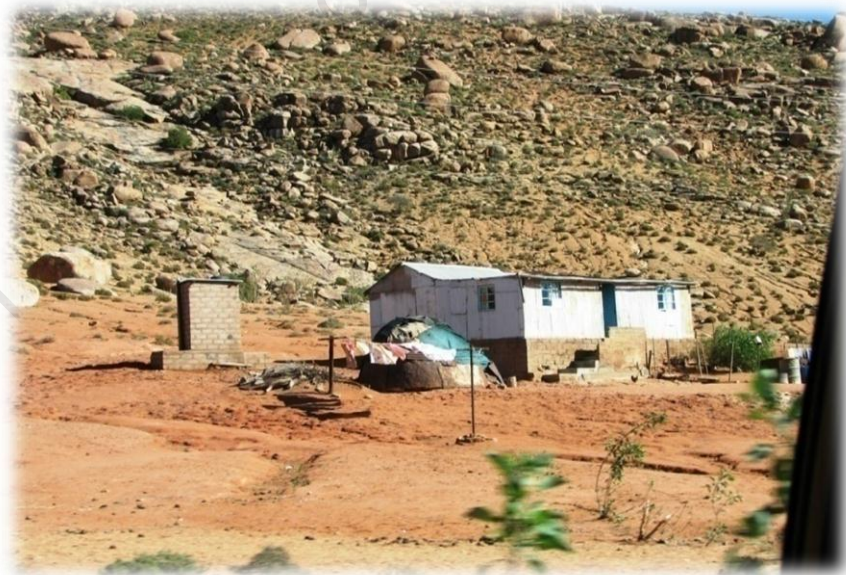
Photograph 2: Outside toilet in Buffelsrivier, Northern Cape.
