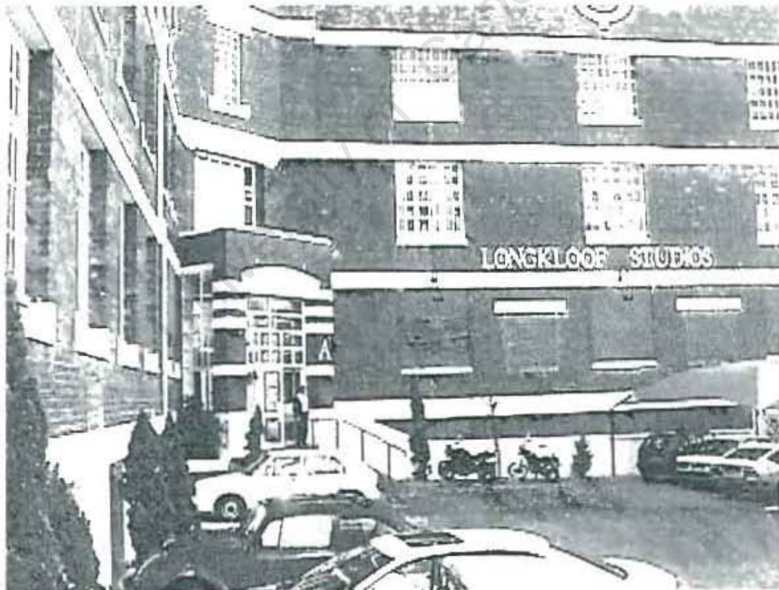
Fig. 24: New entrance between Building 1 and Building 2 (front)
