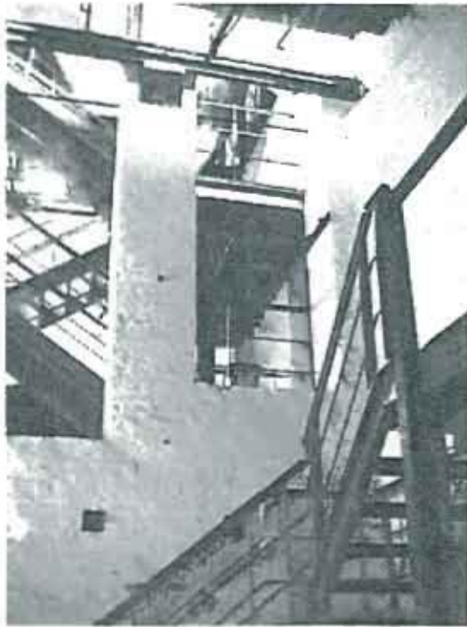
Fig. 37: New staircase (part of visitors' route)
