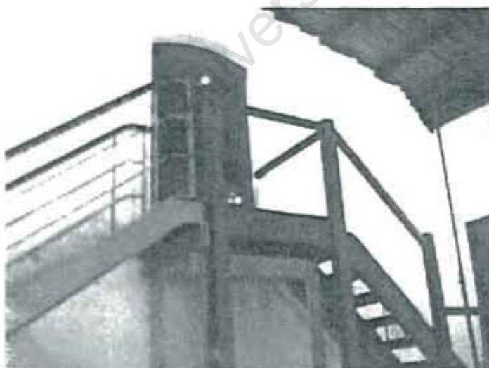
Fig 36. Original staircase and obviously modern new staircase (Mariendahl Brewery)
