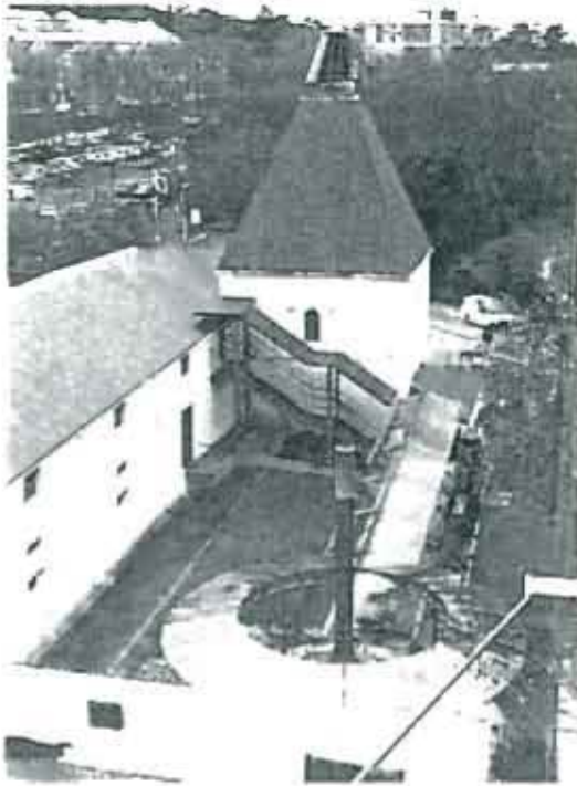
Fig. 32: View of malthouse with kiln as it looks today (top level of Mariendahl Brewery)
