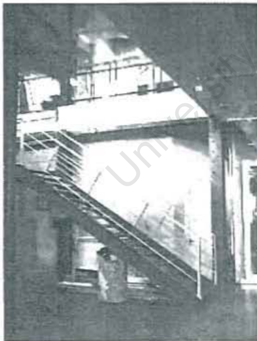
Fig. 25: New staircase in harmony with industrial look of space (Building 2)
