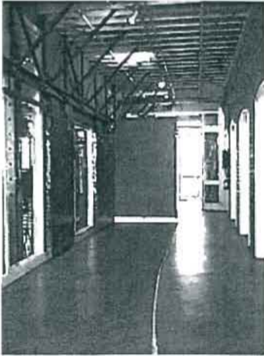
Fig. 26: Passage with wall made of old fire doors (left)
