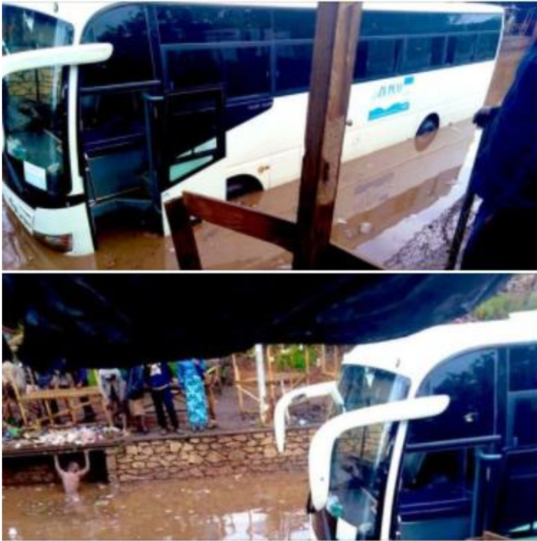
Photograph 10 Condition of transport infrastructure in Harare (Chin'ono, 2021)
