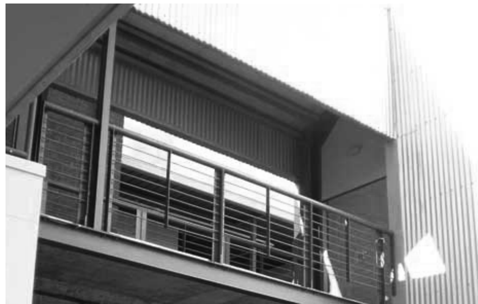
fig 74 (Aragao, 2011): Balcony, upper level
