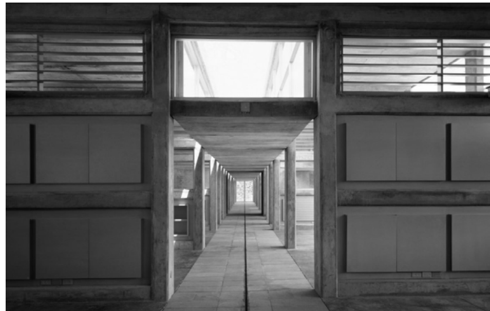
fig 57 (Carrillo, 2020): Different material infill on vertical surfaces between concrete structural frame
