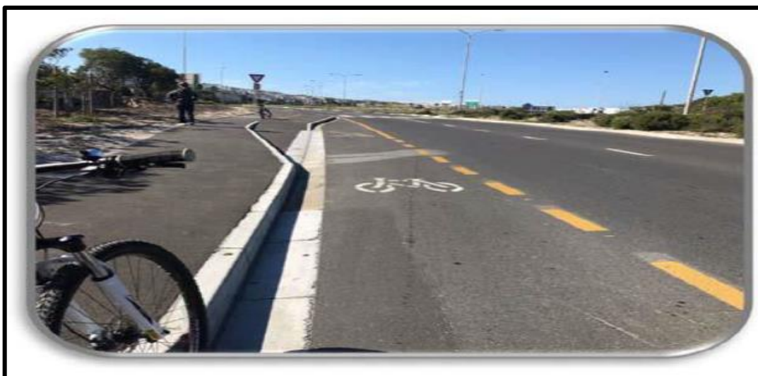
FIGURE 25: BICYCLE LANE DEVELOPED IN EXISTING ROAD SHOULDER (SOURCE: COW, 2018)
