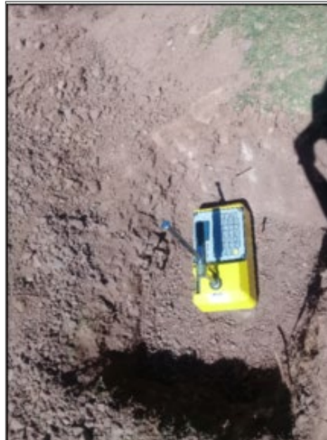
Figure 4-2, Troxler test on site
