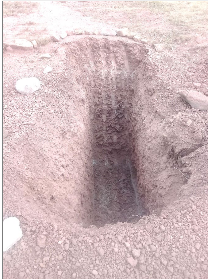
Figure 5, Trial pit 2 (TP03) in Mount Moorosi
