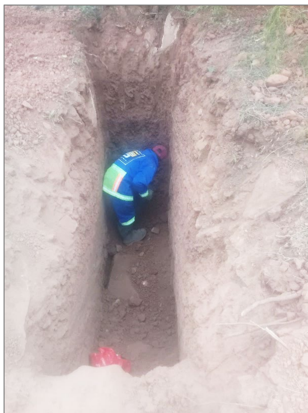
Figure 3, Trial pit 1 (TP01) in Mount Moorosi
