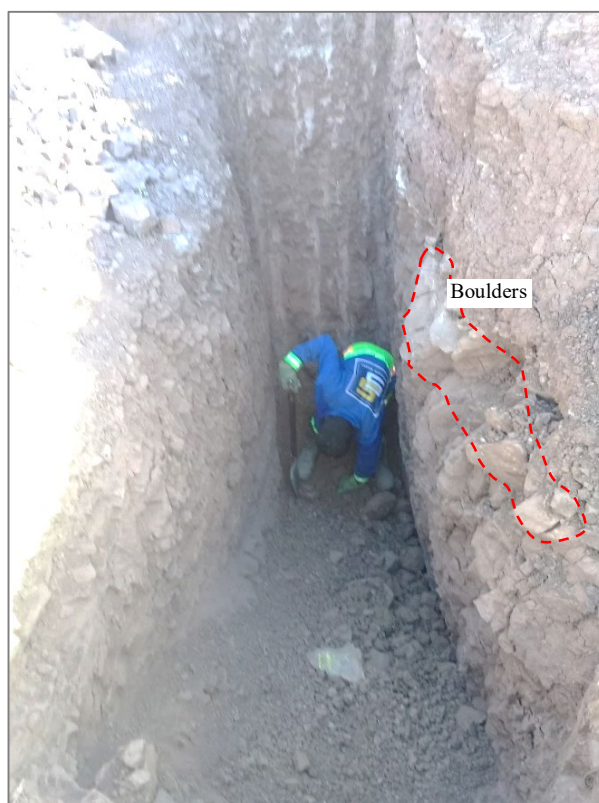
Figure 7, Trial pit 3 (TP03) in Mount Moorosi
