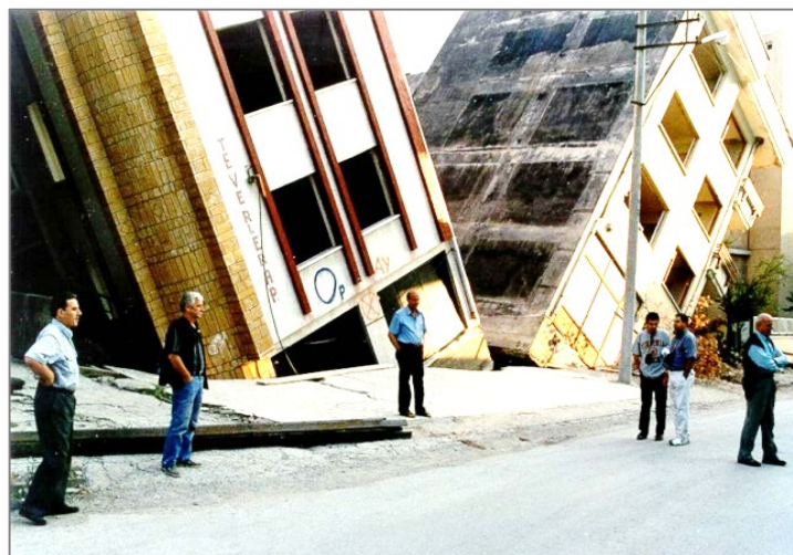
Figure 2-7, Tilting of buildings induced by foundation soil liquefaction in Chile (Source: Bray et al. 2000)
