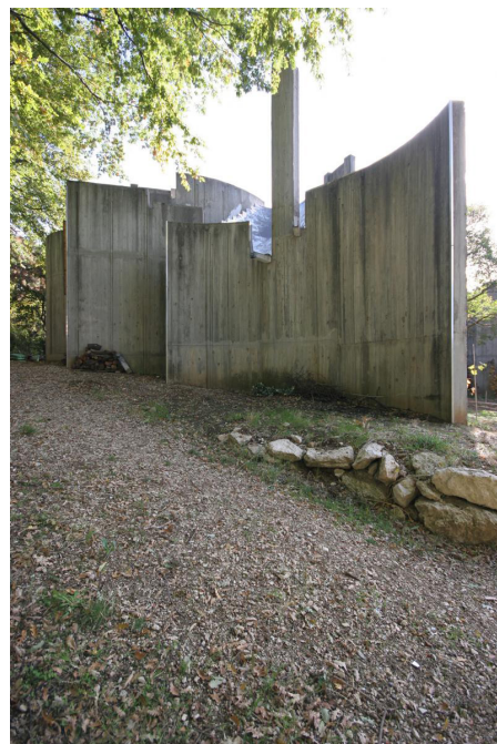
64. Exterior material blending with the ground. source: https://censimentoarchitetturecontemporanee.cultura.gov.it/scheda-opera?id=4056
