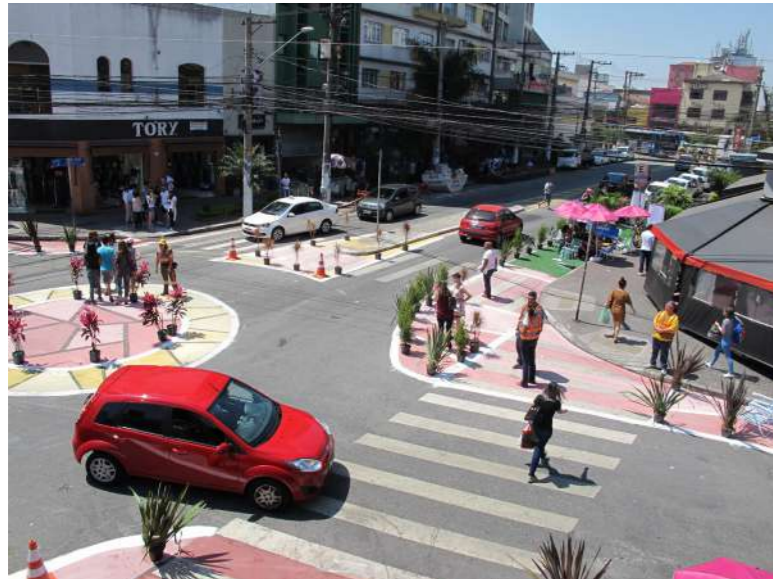
Fig 9.4 Tactical urbanism using painted pedestrian walkways at intersections Source: Global Designing Cities Initiative
