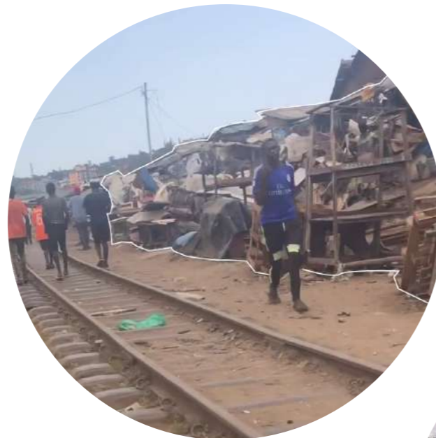
Fig 8.10 Structures demolished in Go-down Zone during an eviction operation Source: Author
