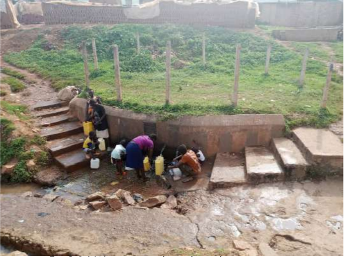
Fig 8.16 Water point along the railway reserve Source: Author
