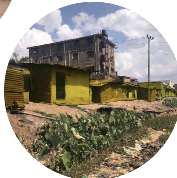
Fig 8.11 New temporary structures close to Go-down Road Source: Author
