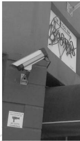
Figure 5.13 CCTV surveillance outside Bronx Action Bar
