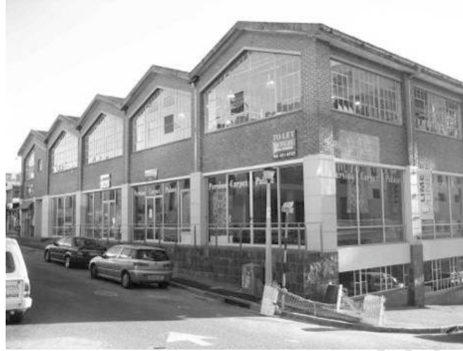
Figure 5.7 Adaptive use: from light industry to retail in De Waterkant, April 2007
