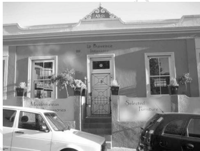
Figure 5.8 Adaptive use: from residential to retail in De Waterkant
