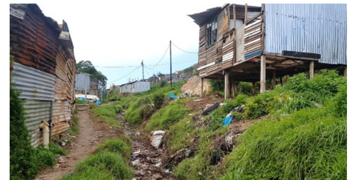
Figure 2.9: informal structures (Source: author)
