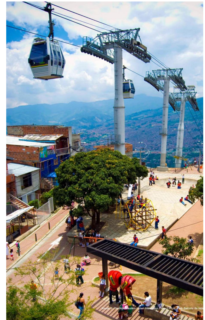
Figure 3.10: EL Mirador Park in Medellin (Source: https://issuu.com/dannyandresosoriogaviria/docs/the_northeastern_urban_integration_ )
