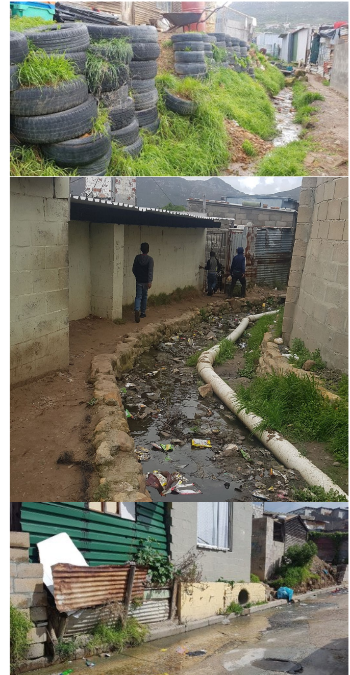
Figure 4.8: Water systems in Hangberg (Source: author)
