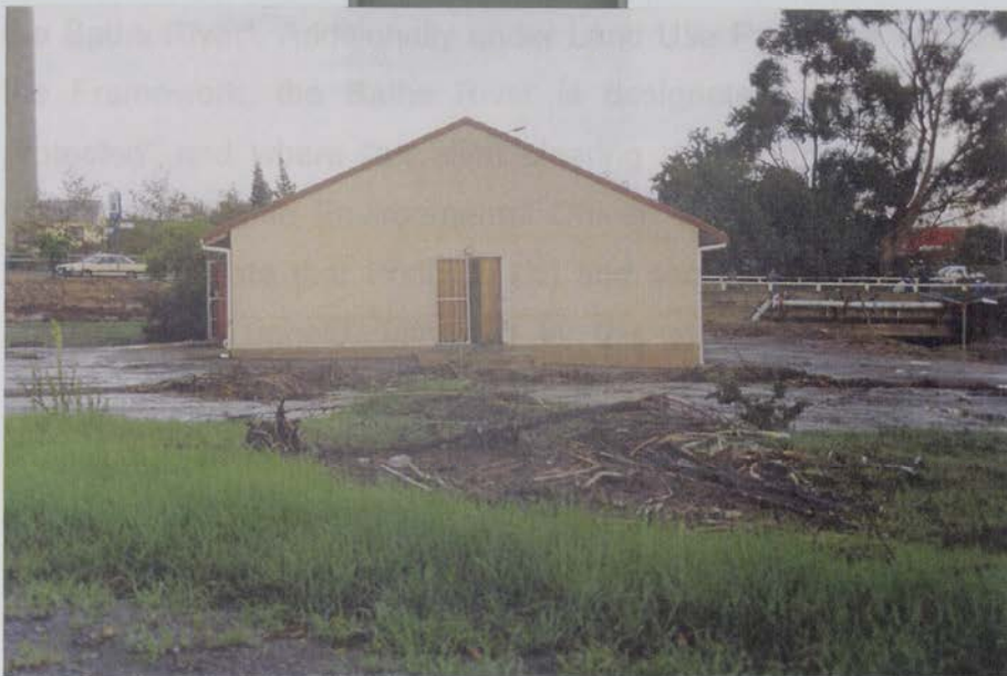
Figure 5.2: The Caledon Clinic post April 2005 flooding event
