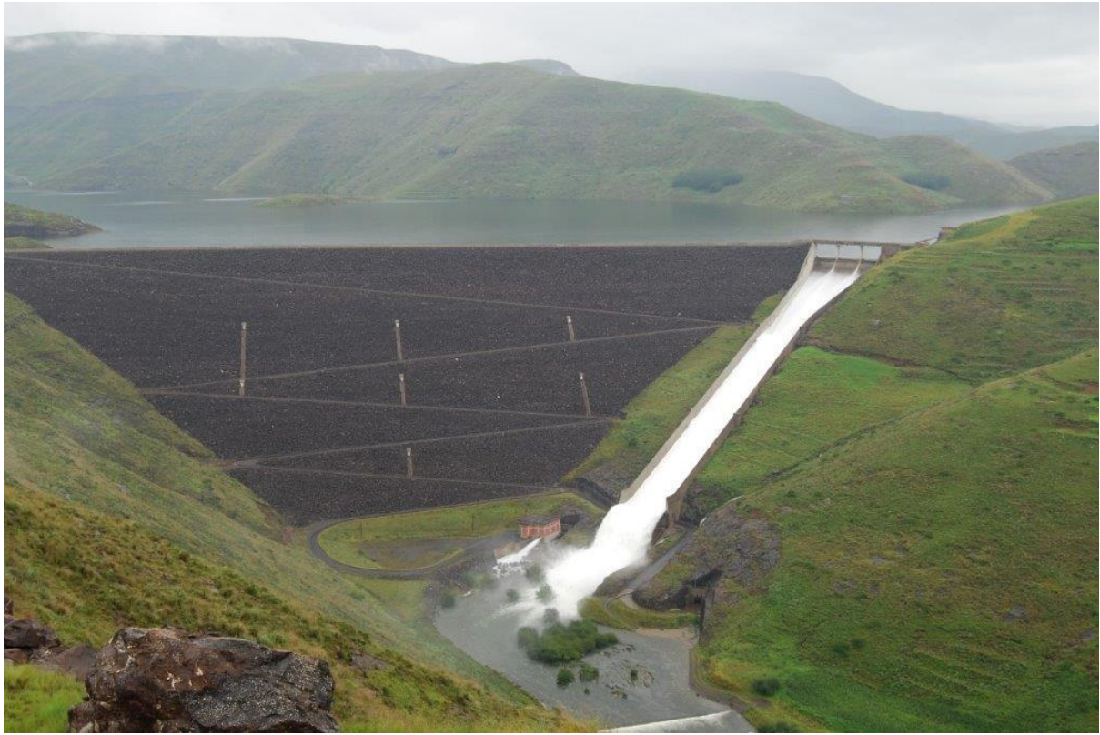
Figure 3 Aerial picture of the Mohale Dam. Source: LHDA 2016
