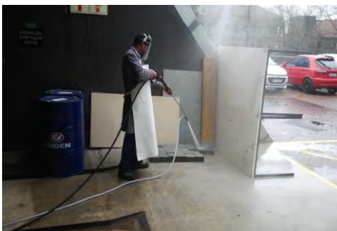
Figure 3.16: wet sandblasting
