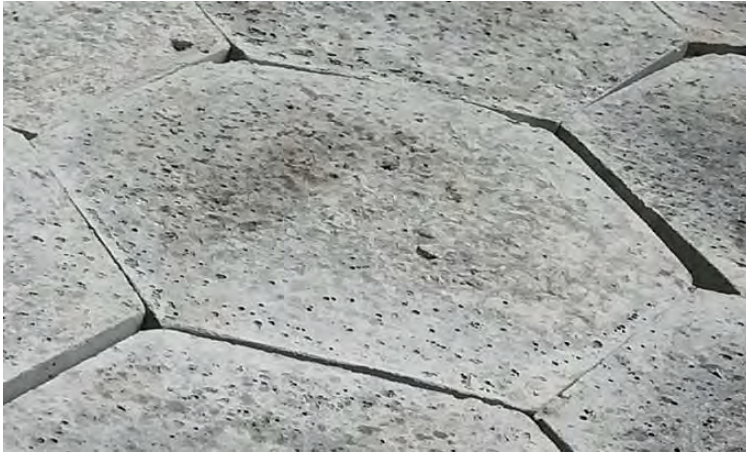
Figure 3.19: substrate surface prior to sandblasting
