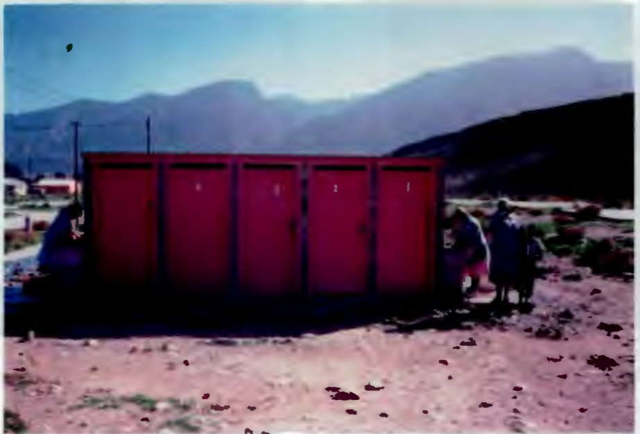
Plate 5.2.: Five toilets serve the 2000 (mainly) seasonal farm workers living in Epukumleni
