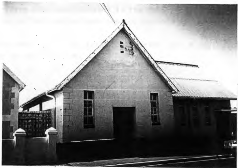
Original entrance from Park Road. The section on the right is a recent extension.
