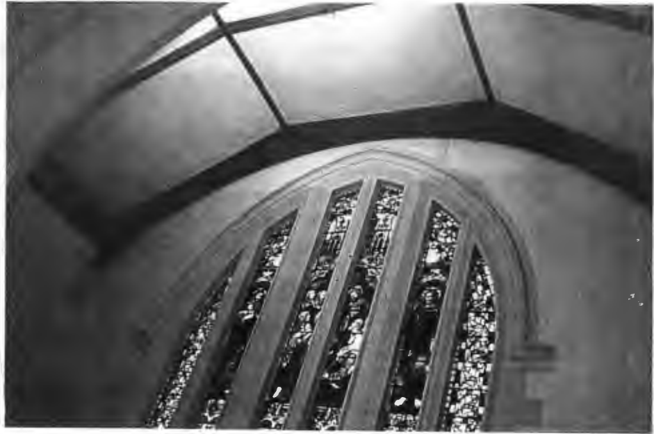
ABOVE: Roof trusses in the right transept; note the shallowness of this element.
