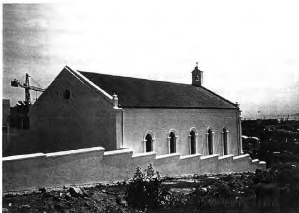
East wall of nave; looking north
