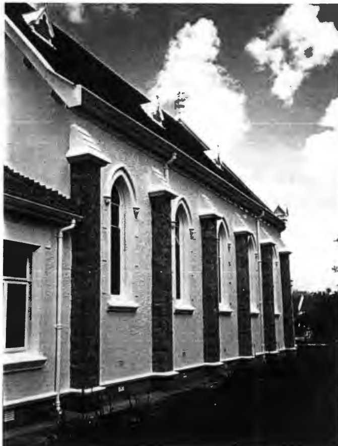
Six straight stone buttresses on nave wall.
