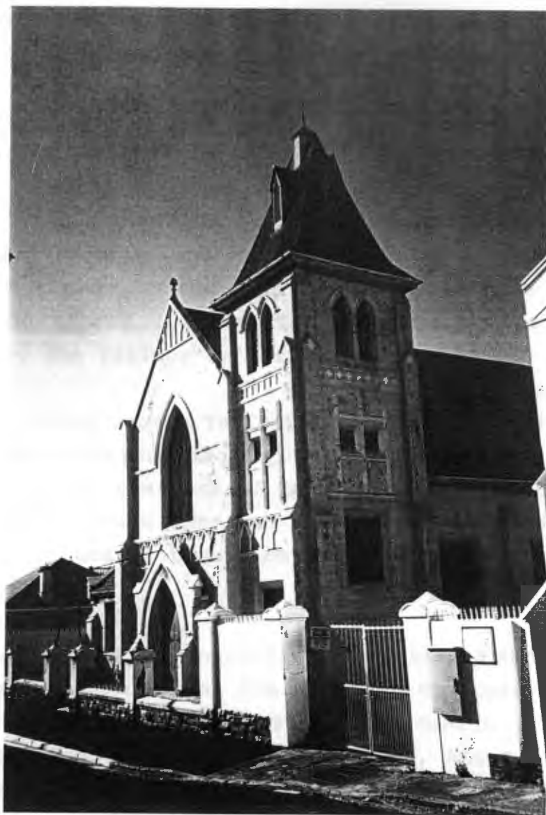
Note use of both pointed and flat-headed windows on nave gable-end wall and side wall of nave.
