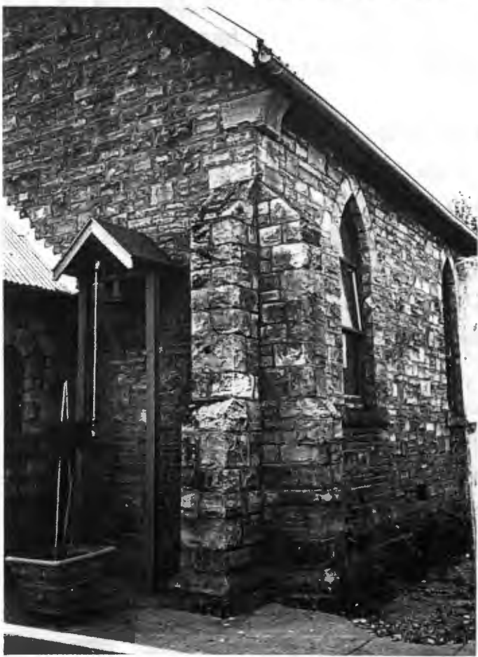
ABOVE: Angle buttresses and curved sandstone block at base of gable.
