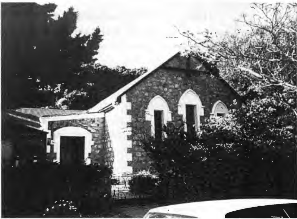
Entrance from Main Road
