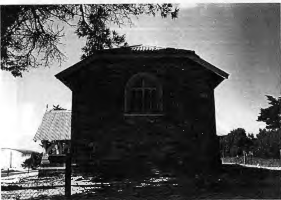
View from north showing end wall of nave with its hipped gable roof.
