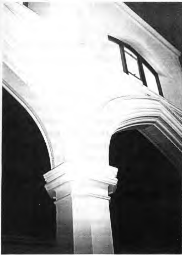
LEFT: Octagonal columns and pointed arches in the nave.
