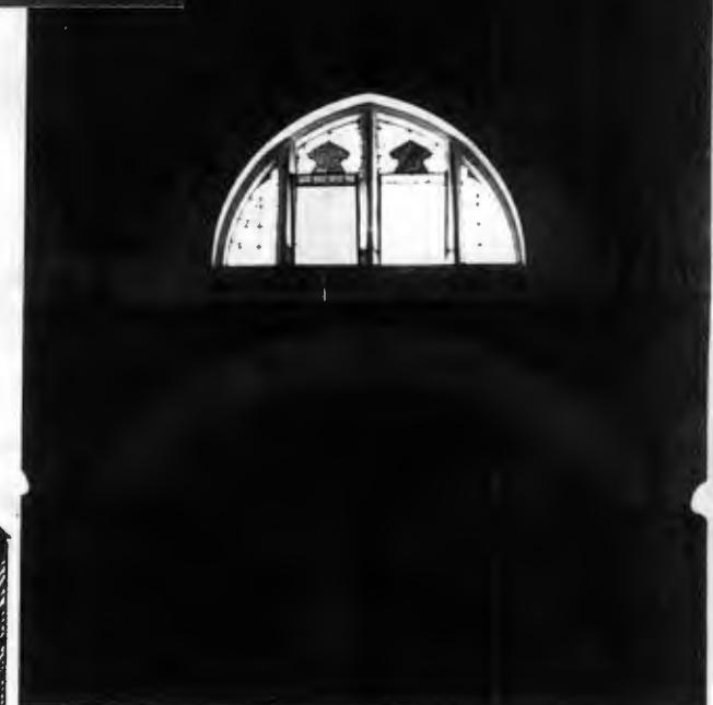
Clerestory window and aisle arch
