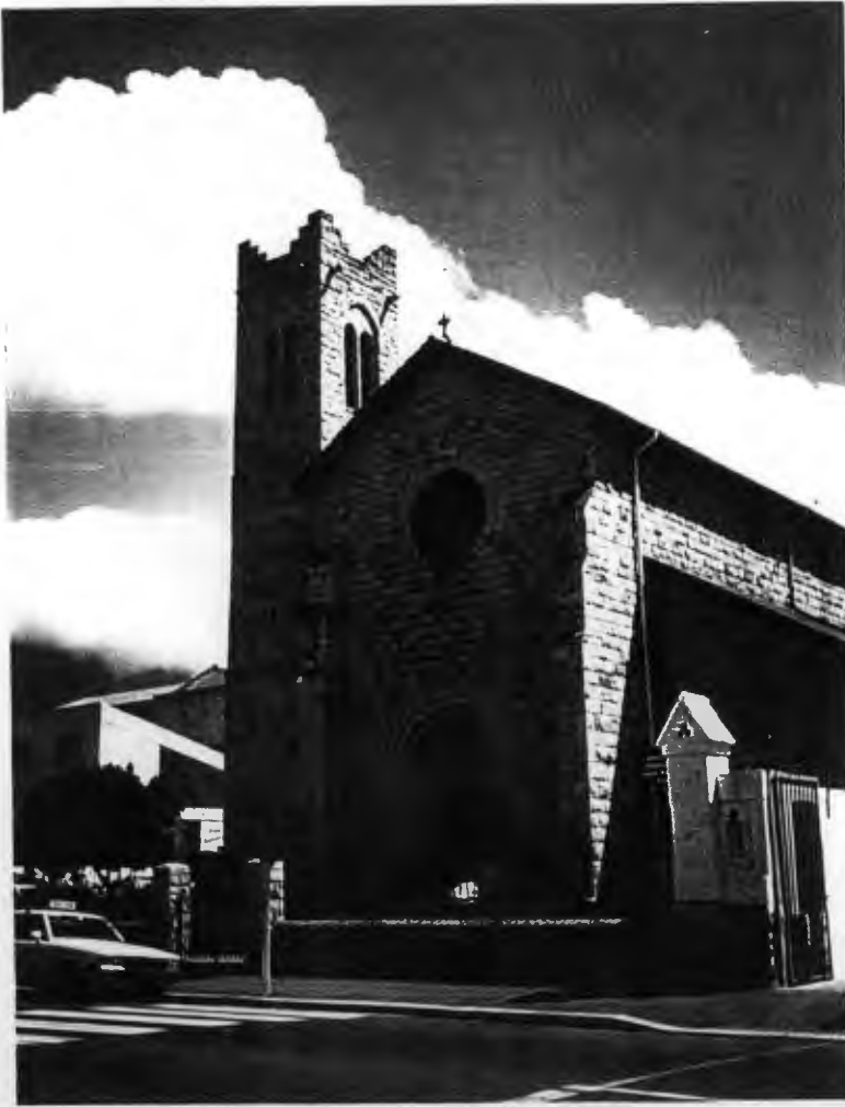
Impressive basilica in the Italian style, fronting Somerset Road Note three-step buttresses, high clerestory windows and recessed entrance.
