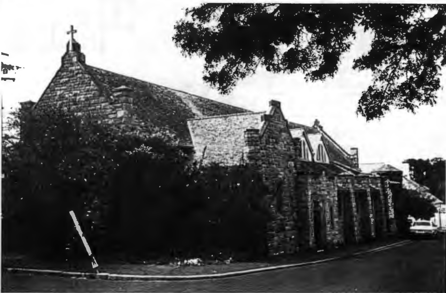
Apsidal end; south aisle from South-west
