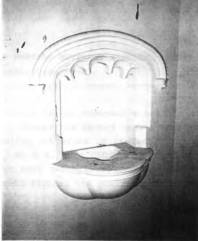
LEFT: Piscina (drain) in apse
