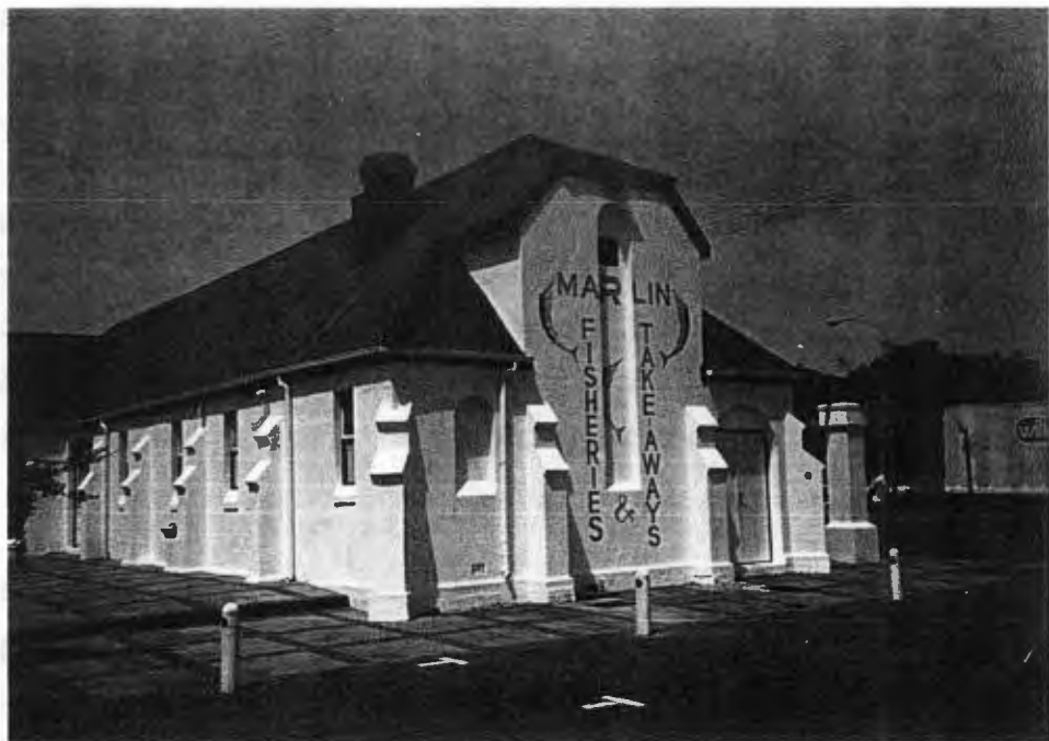
West wall showing unusual roof design, : two-tier buttresses
