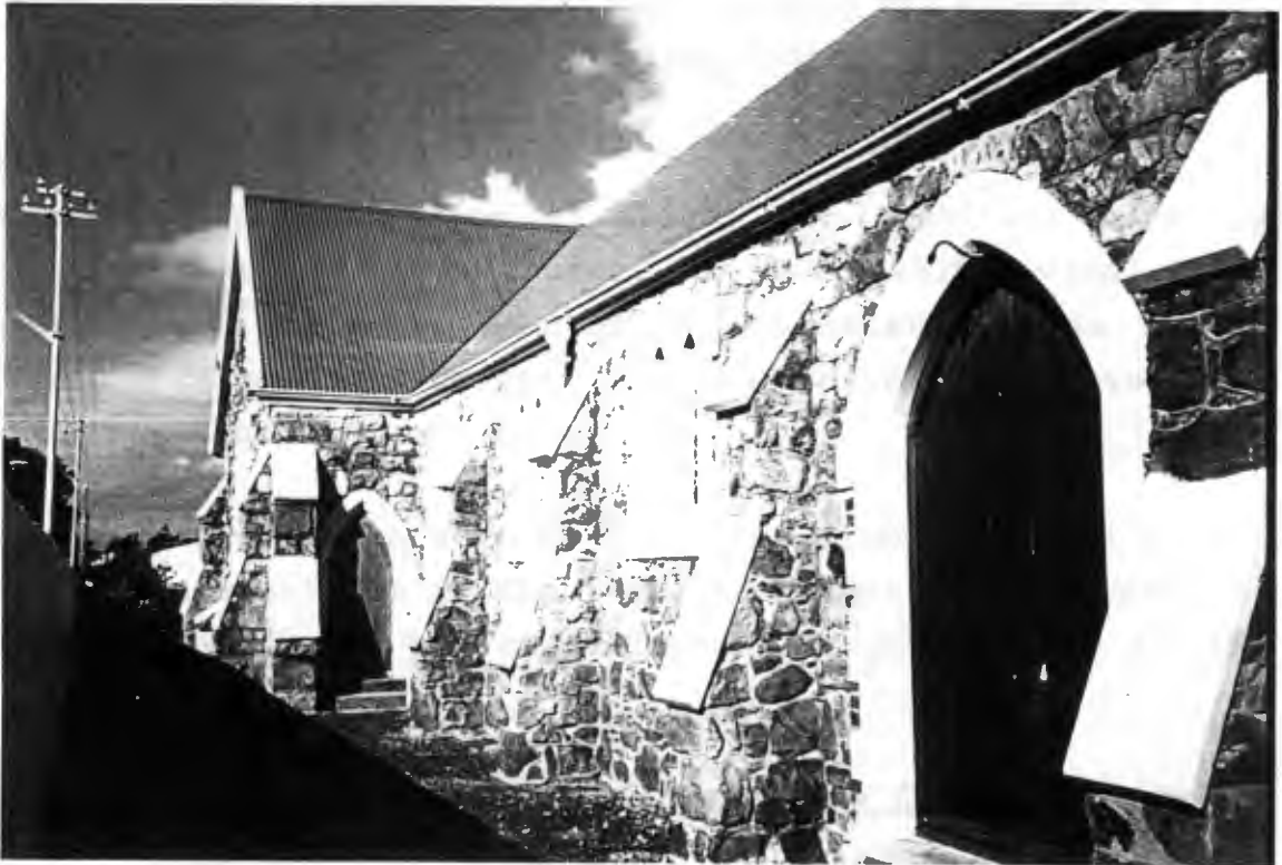
North transept and north wall of nave showing unhewn stonework and two-tier buttresses.
