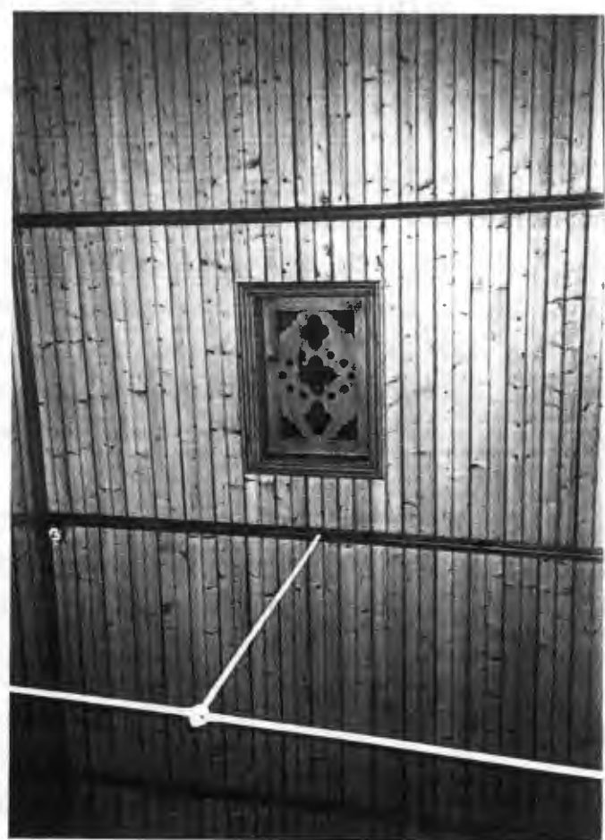
BELOW: Ventilation panel in ceiling
