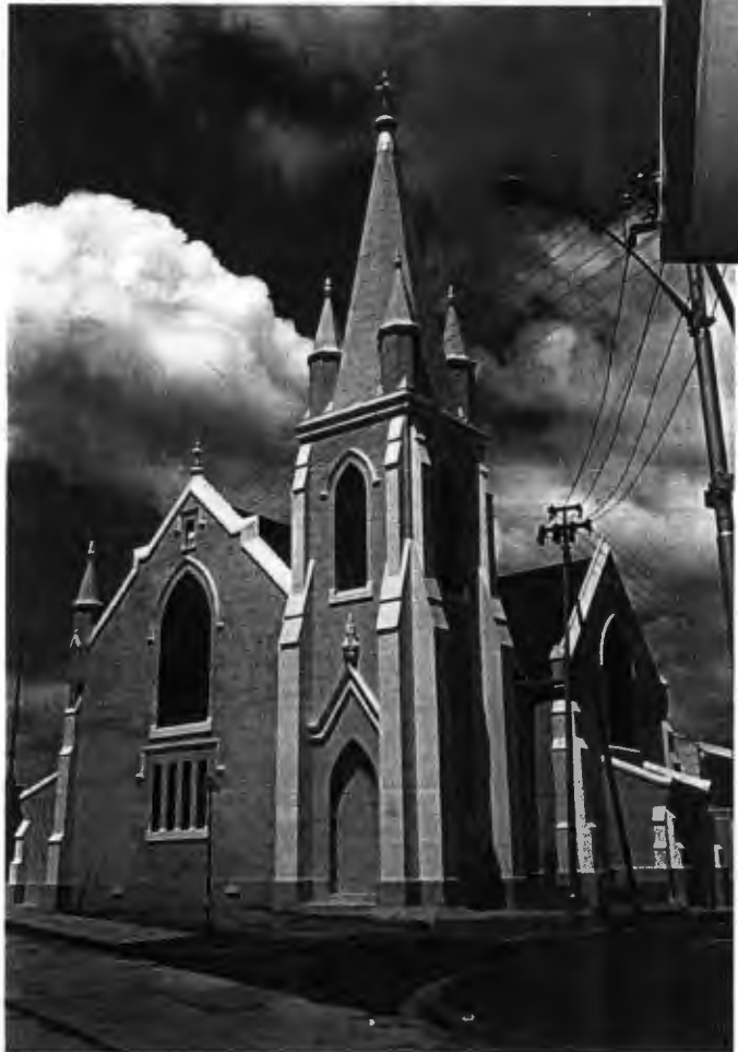
East wall of nave, tower and North transept
