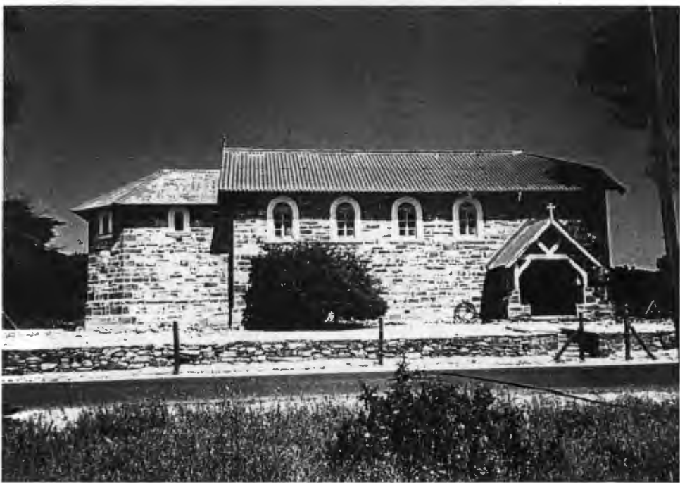
View from east showing apse, nave and timber porch
