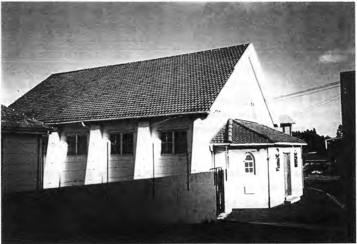
Observatory Baptist Church. Note single tier sloping buttresses and the altered vestibule. One of the two foundation stones is below window.
