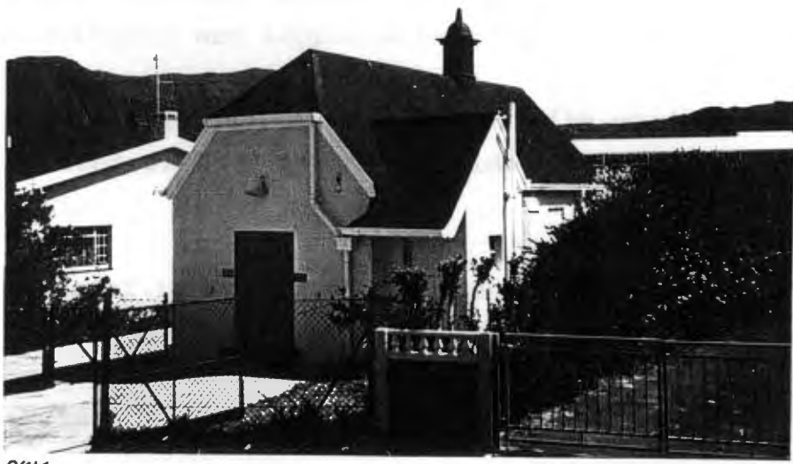
LEFT: East wall showing hipped gable roof, original entrance porch and the ventilation turret.
