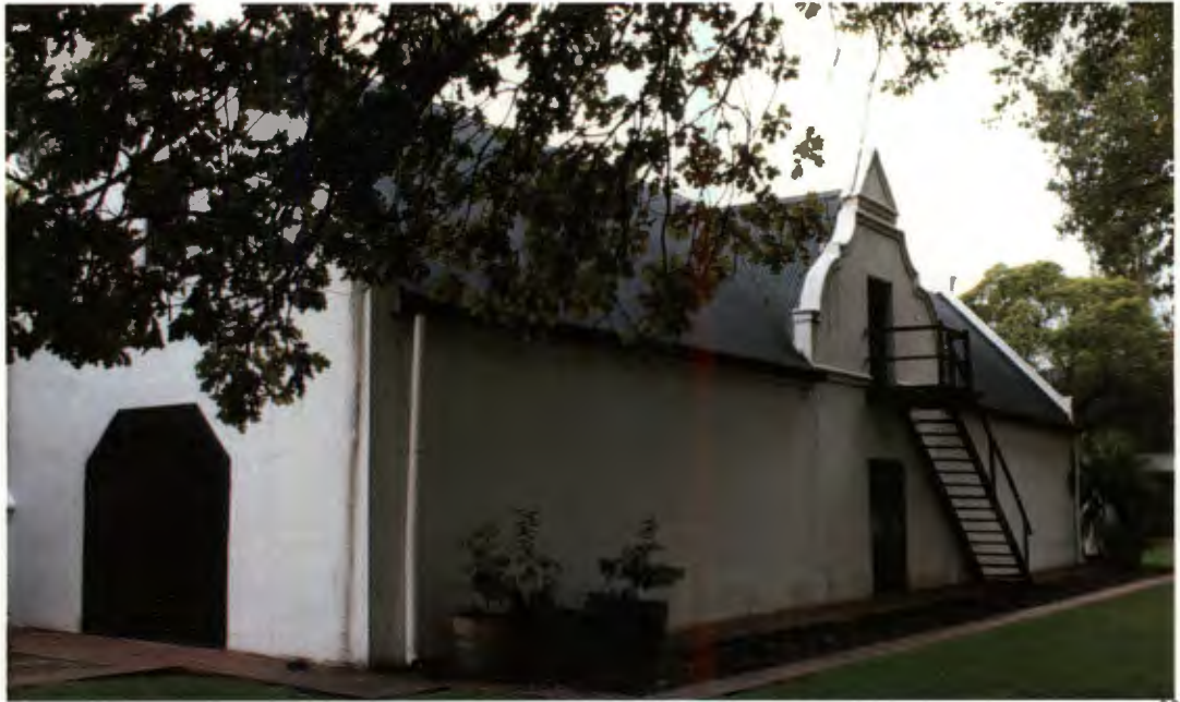
FIGURE 22: An outbuilding on Kanetvlei - the outbuilding and main house were often very similar, as is evident in this photo. The roof is no longer thatch, due to the fire hazards in the region.
