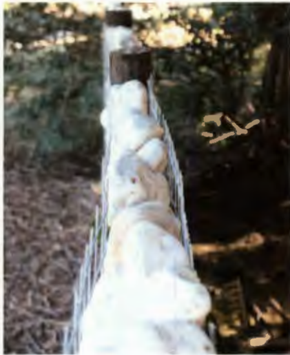
FIGURE 48-50: A 'makeshift' wall: a simple solution. It has direct connection to the ground - no protective measures, and old bark meets the stone at the base. The gum-posts protude above the rest of wall, whether intentional or not, it creates a sense of hierarchy and definition.
