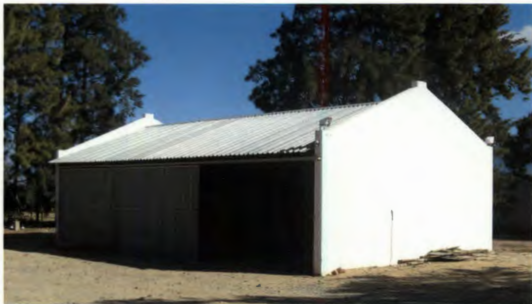
FIGURE 51a: A pseudo steel shed. The steel framed shed ends in whitewashed masonry end gables - it is as if the prefabricated elements are contained by the vernacular. The logical and common fact that a steel frame structure has modular grid is of minor detail here - the grid spacing is inconsistent.
