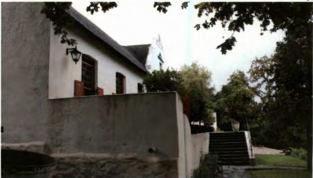
FIGURE 24+25: The stoep at La Plaisante. Figure 13 focuses on the slate/mountain stone paving common on stoeps. The steps were a necessity, to bridge the gap between the stoep and uneven ground. The raised wall at the end of the stoep (fig 14) holds the end bench. This fig. also highlights the uneven white-washed walls, and the stone base that most buildings had.
