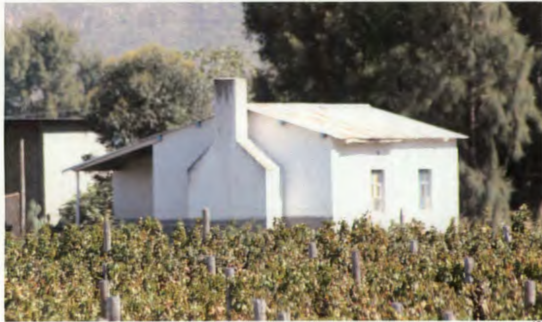
FIGURE 10+11: A white cottage with its komyntjie. The symmetry and proportion of the cape vernacular is illustrated here. Furthermore, this illustrates how the cottages sits in the vineyard - set amongst the vines, only the top halves of the cottages stick out, and they appear like white floating elements in a sea of greens, reds and browns.
