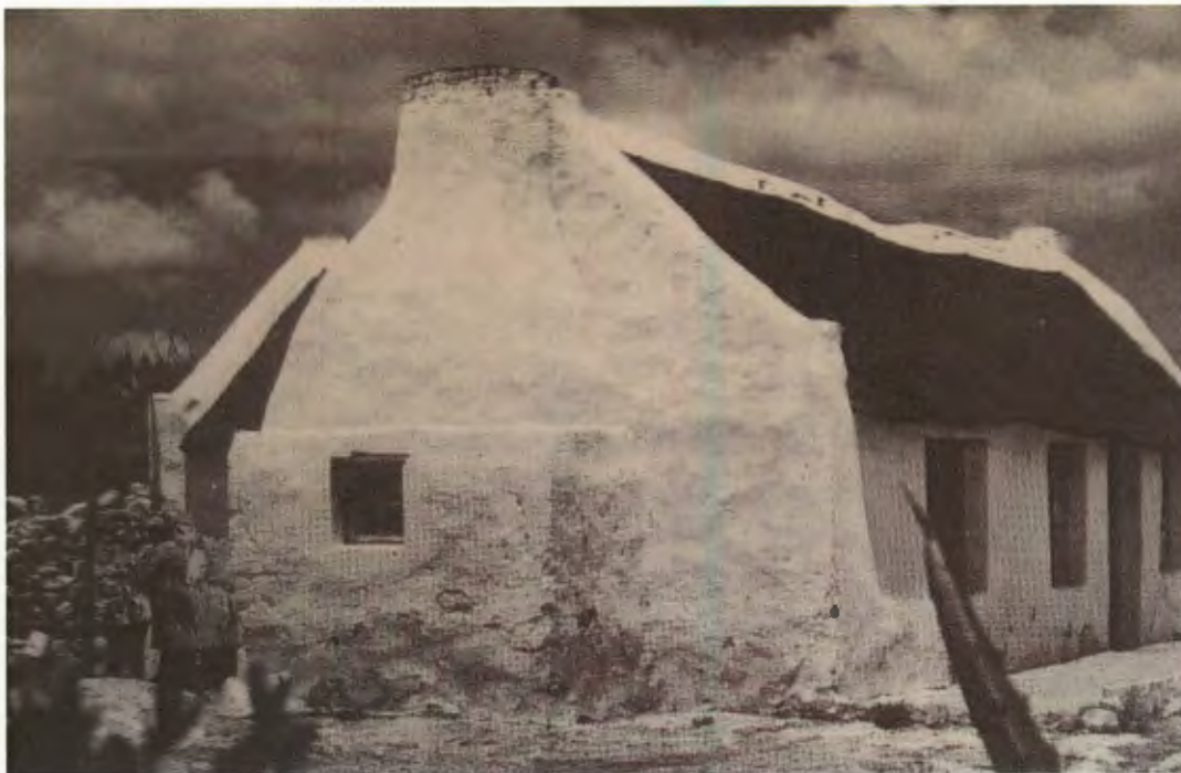
FIGURE 29: Cottages and their komyn-tjies. Despite being in different regions, all these cottages typify the 'komyn-tjie' element, and its resultant sculptural feature. This is an element that is still evident in the farming communities in the Breede River Valley for example.
