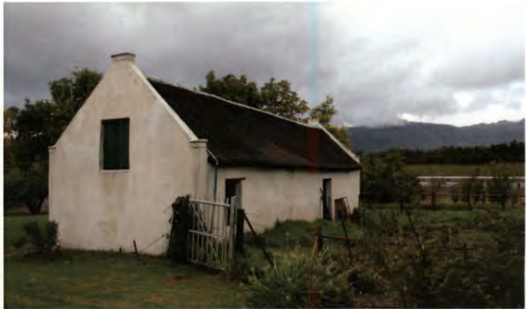
FIGURE 23: An outbuilding on La Plaisante farm. The simplicity and uneven whiteness of the end gable creates a moment of pause in the busy landscape. The mock chimney at the top of the gable is a typical characteristic, as is the door which allowed access into the loft. The parapets of the end gable extend above the line of roof to form a buffer against the wind. Another typical feature is the coping at the apex of the thatch, which was also a protective measure.
