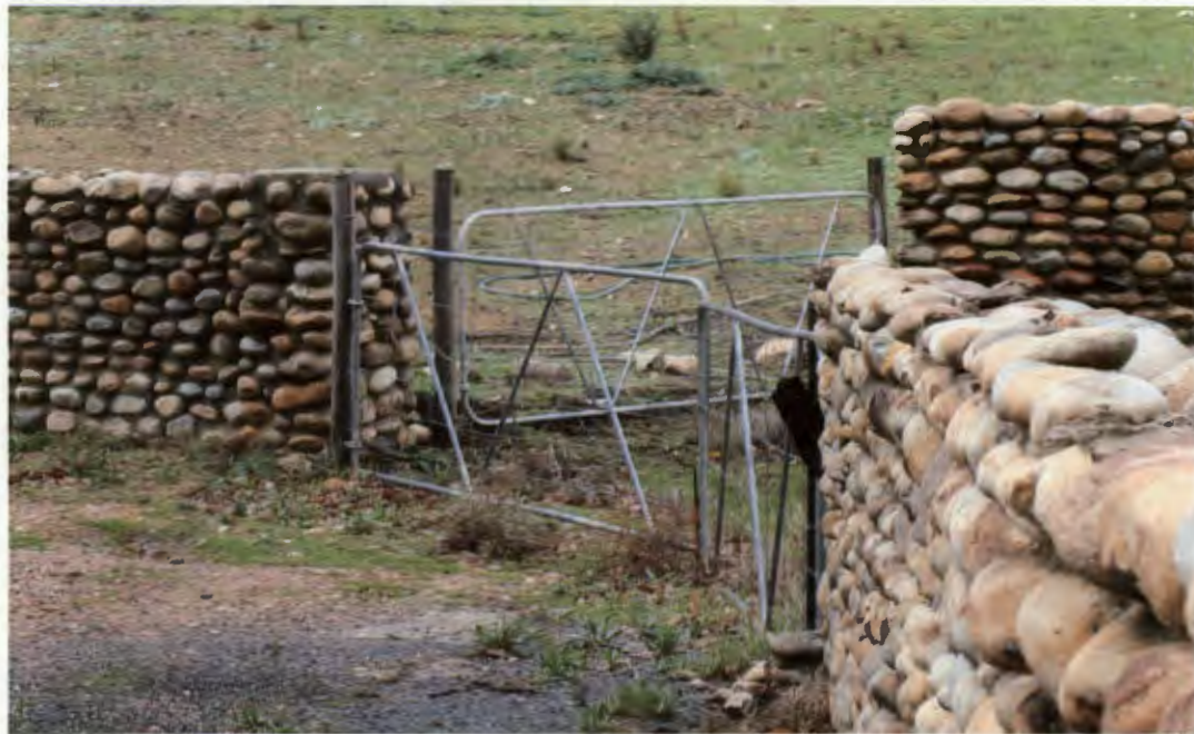
FIGURE 42: A stone wall used to create paddocks/fields on a farm. The stone is neatly packed in rows (with a preference for flatter shaped stones for easier construction), displaying a variety of colours. These colours resonate within the context and so the walls tend to blend in with its surroundings. To contrast the localness of the stone, the mass produced, off-the-shelf metal farm gates hanging on a gumposts become the opening and the 'light' elements amidst the solidness of the stone.
