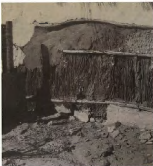
FIGURE 28: Cottage at Oudekraal fontein. This image shows the construction detail - timber vertical wall posts and horizontal laths supported reeds which acted as 'infill', and this was then plastered with lime. The boen-onder door is another characteristic element found all the Cape vernacular - it was functional as it could let light and air in with the top half open, but animals and children could be controlled by the closed bottom half.
