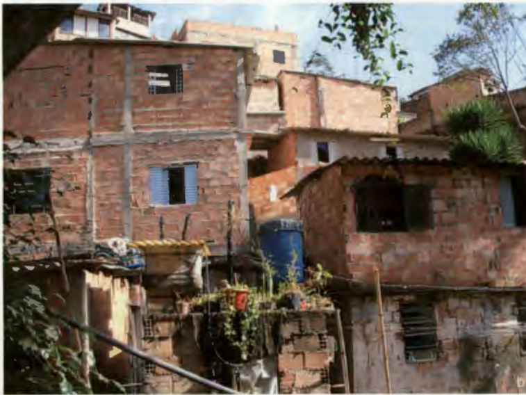
FIGURE 9: an illustration of modern technical tenets appropriated by the favelas. a-b. favelas in Belo Horizonte: a rudimentary interpretation of the concrete post and beam system forms the basis of the structural system in the working class neighbourhoods. The easily accessible concrete and the willingness to have a 'vernacular' technique of formwork has lead to this technique as disseminated across society, to all building types..
