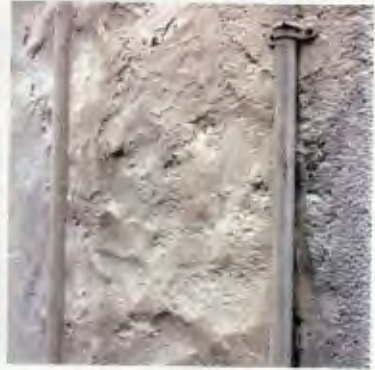
A rough texture - an old wall.
