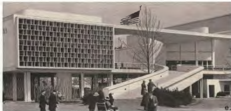
FIGURE 7: the brise-soleil: different forms of sunshading devices as a modern tenet. a. blocks of apartments in Rio de Janeiro - here is a variety of sunshading devices: awnings and shutters; b+c..Day Nursery, Gavea, Rio de Janeiro by Niemeyer - adjustable vertical asbestos blinds. Not only does it protect from the shade, but it also creates an varied facade dependent on the position of the blinds; d. The Ministry of Education and Public Health, by Niemeyer. e+f. Brazilian Pavilion, New York World's Fair (1939) - another application of a brise-soleil version to project a glass facade.
