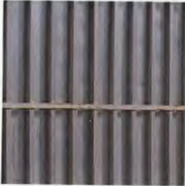
Corrugated sheeting - shed doors
