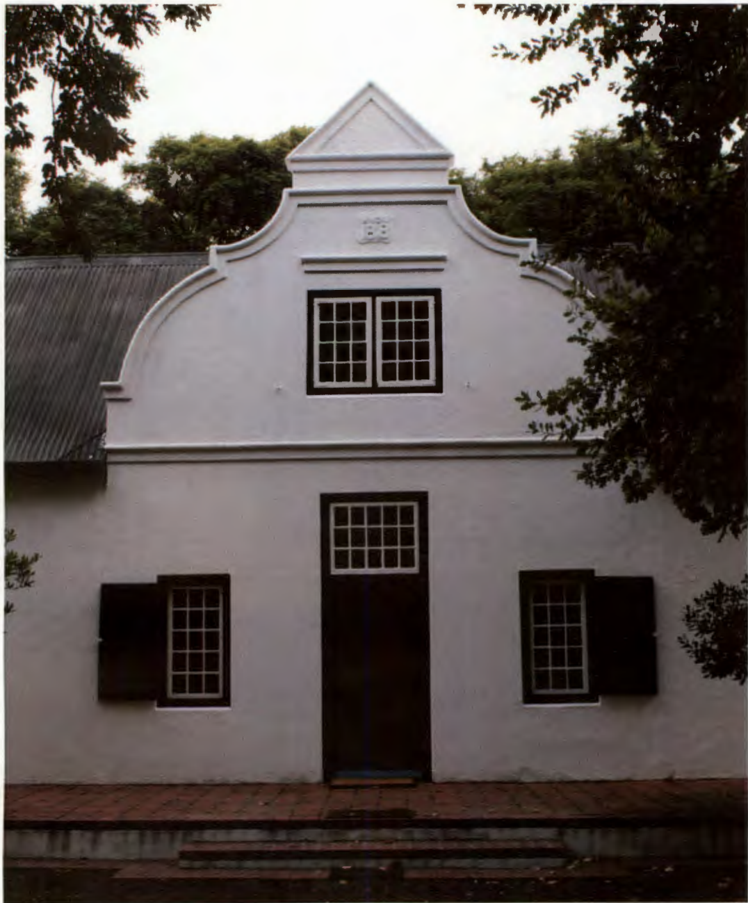
FIGURE 20+21: Front facade of the main homestead on Kanetvlei Farm, Hex River. The entrance door is placed symmetrically in the centre of the gable, and thus, being protected by the gable, the inhabitants could run out in the case of a fire (the burning thatch would fall against the back of the gable).
