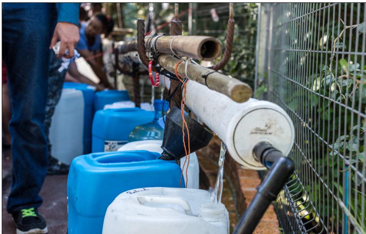
Fig. 16. Riyaz Rawoot's improvised pipe structure helping more people access the water commons at Springs Way Spring. Image: Sid Lockett. 2018. 160
