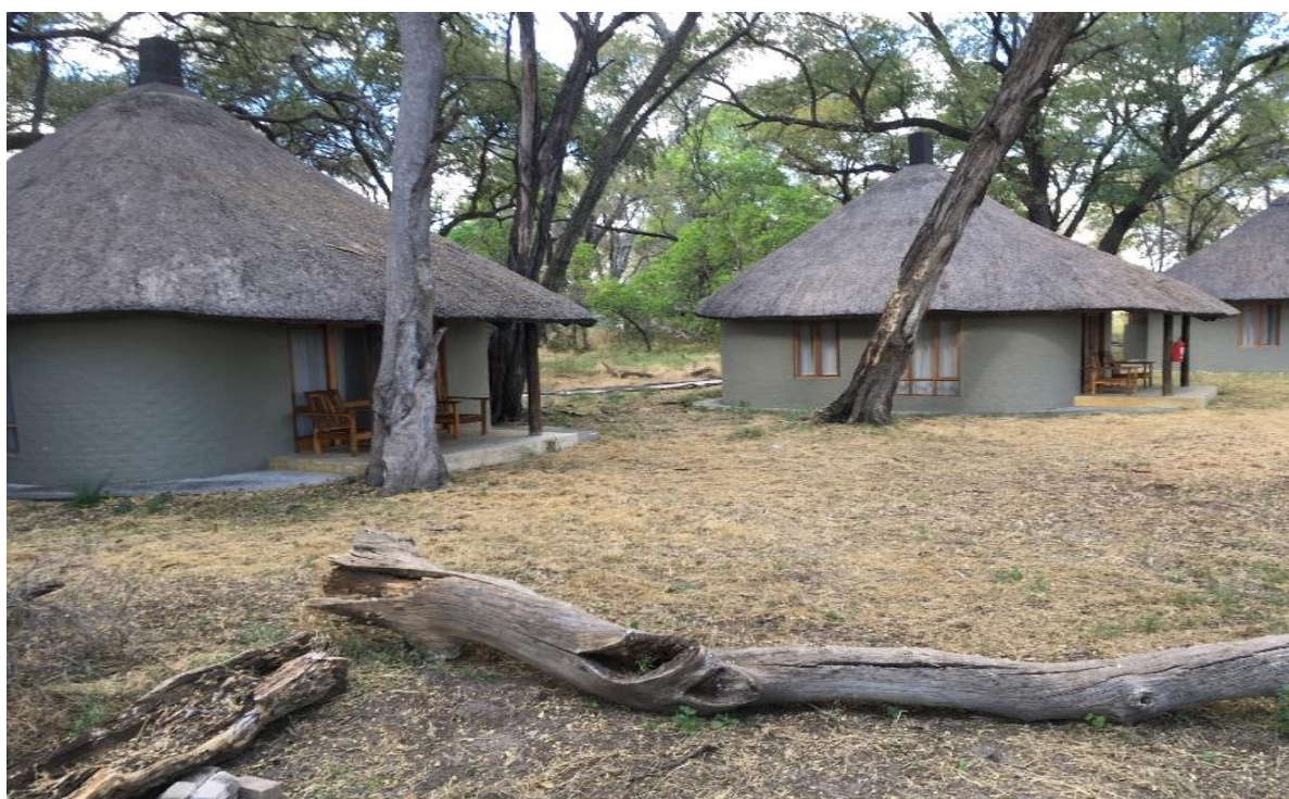
Figure 6.7: Tsaro lodge Chalets built with brick and mortar (Source: Author, 2018)
