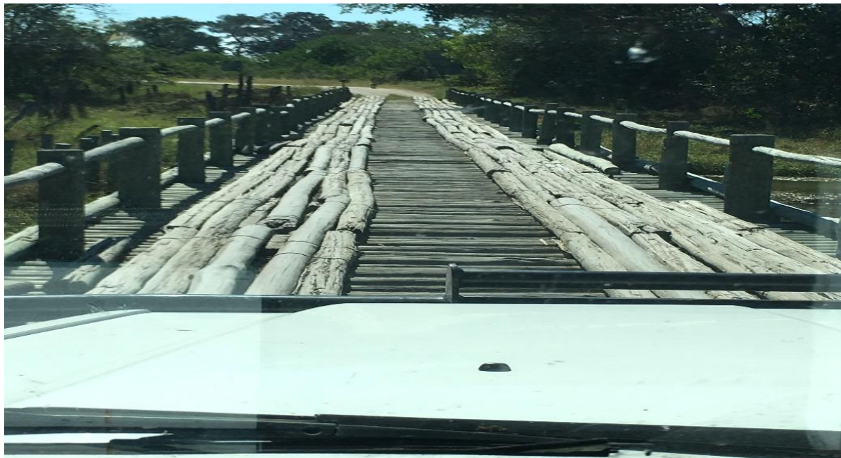
Figure 6.2: Wooden Bridge in a community concession (Source: Author, 2018)
