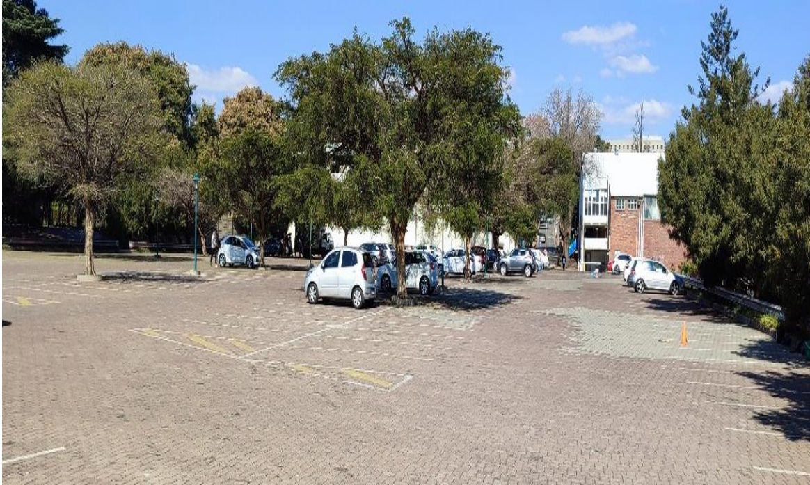
Figure 6-4: Trees can significantly increase clogging in PICP
