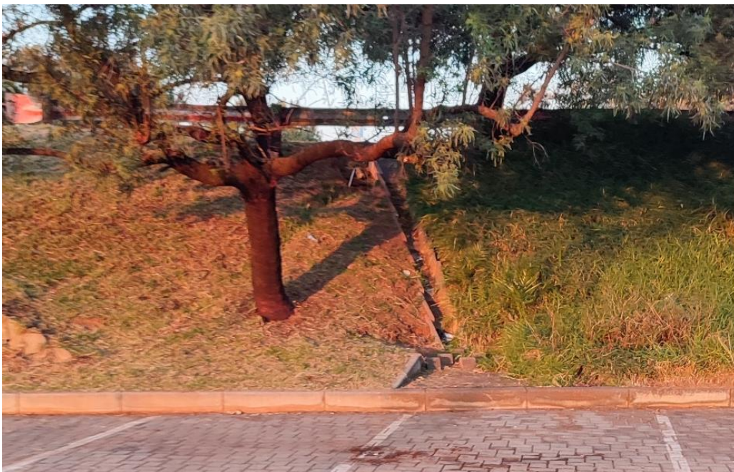
Figure 4-101: Typical concrete-lined chute between WITS-U and WITS-L
