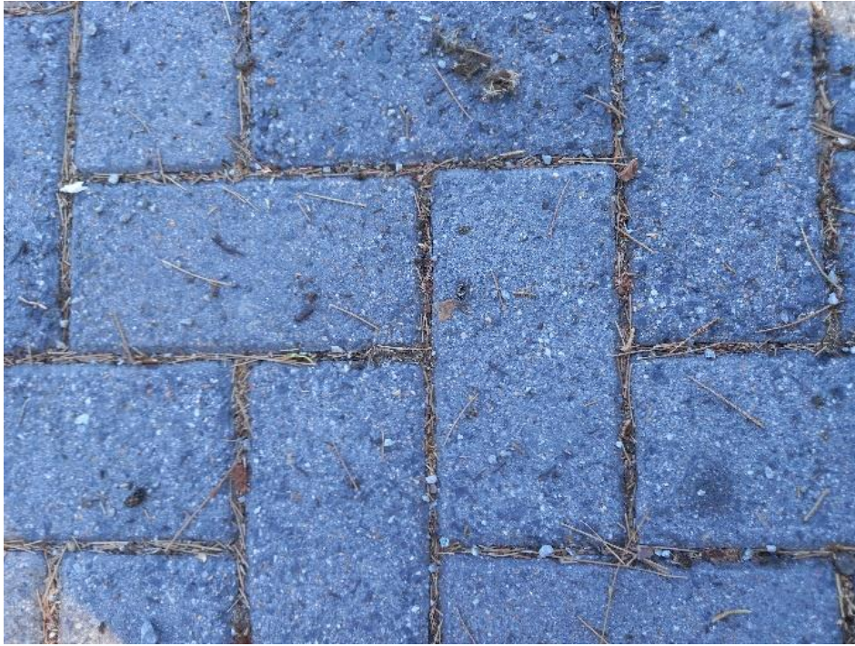
Figure 4-12: Typical PICP section with needle-shaped leaves wedged in the joints
