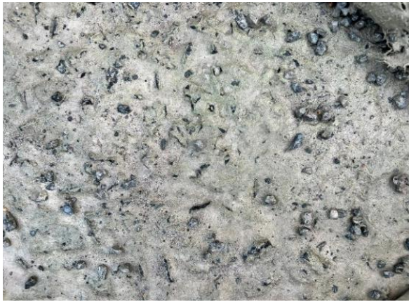
(a) NEB-04 state of the geotextile
