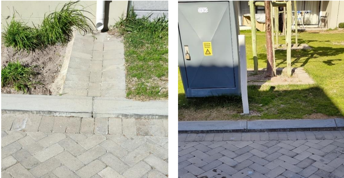
(a) Downpipe and vegetated strip
