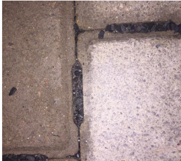
Figure 5-15: Typical sediment accumulation between the Aquaflo ® pavers
