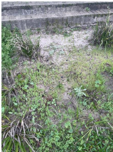
(a) Sediment source adjacent PICP
