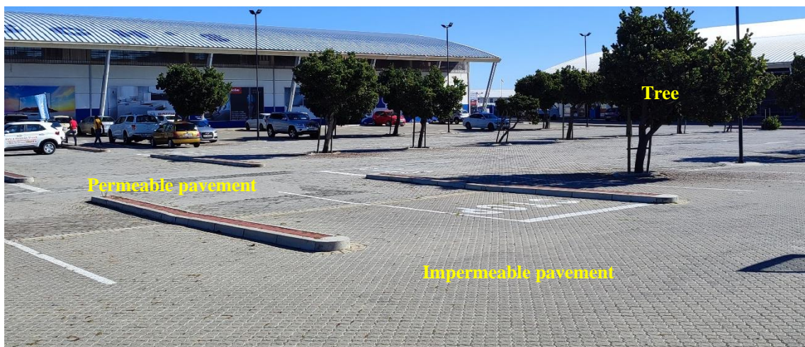
Figure 4-80: HAM PICP permeable and impermeable pavements, and tree distribution
