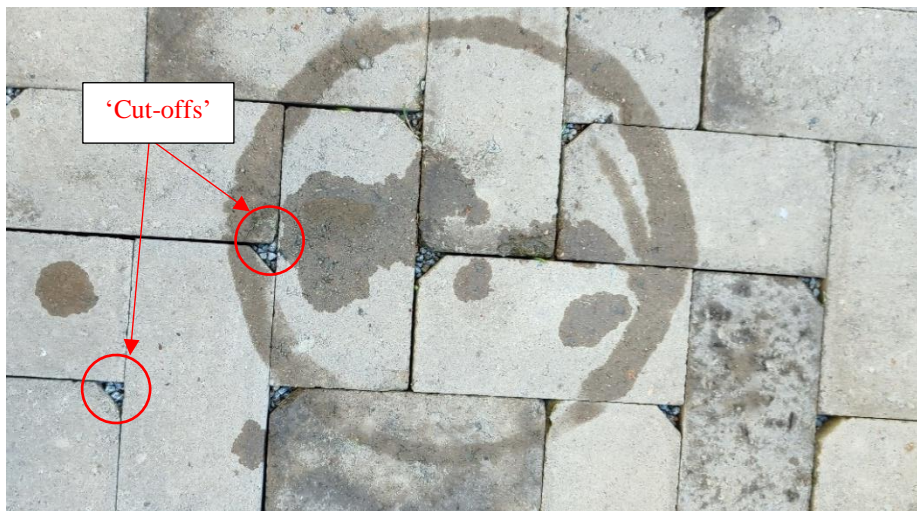
Figure 4-92: Typical 'cut-off' pavers
