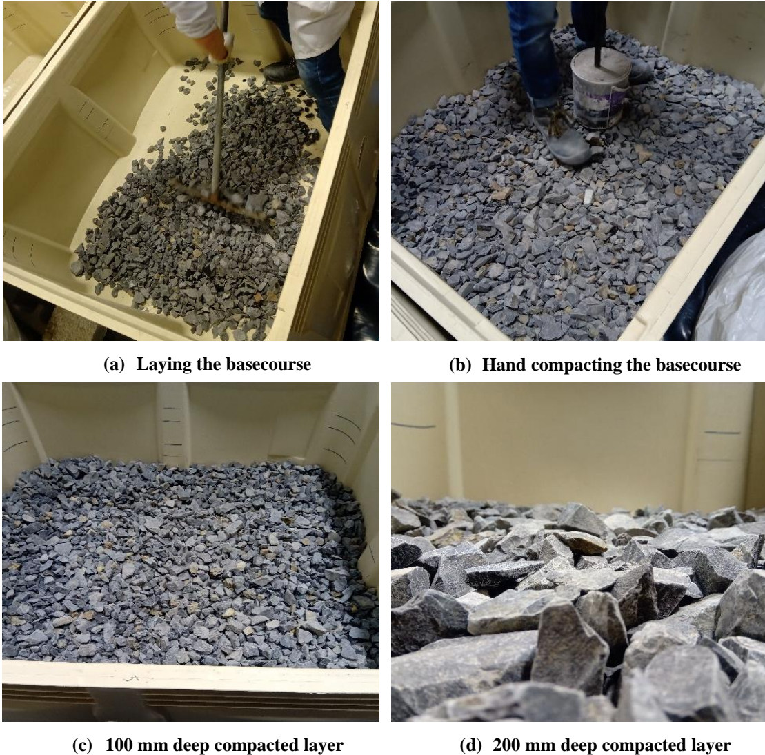
Figure 5-4: Construction of the basecourse layers in the experimental cells
