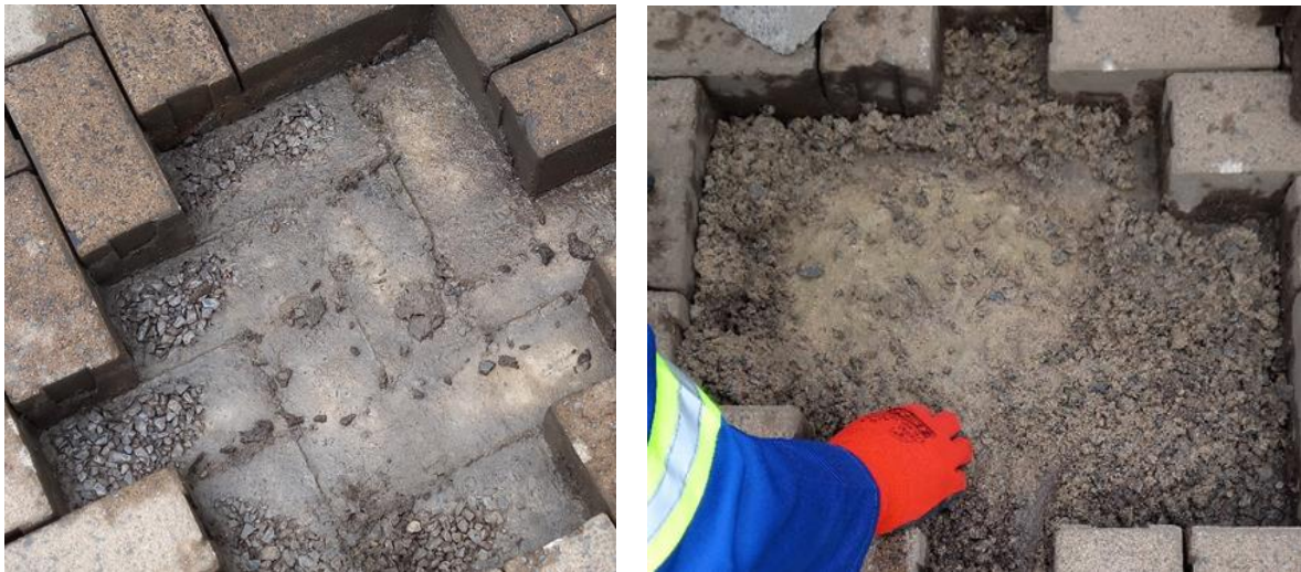
Figure E-3: Type III clogging (of the bedding)
