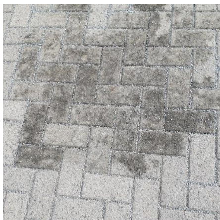
Figure E-7: Repaired PICP test spot
