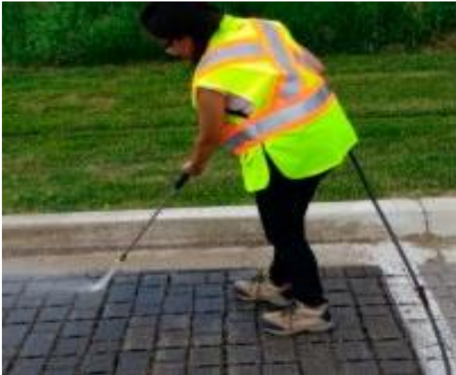
Figure 2-33: Water jetting (Sehgal et al. , 2018)
