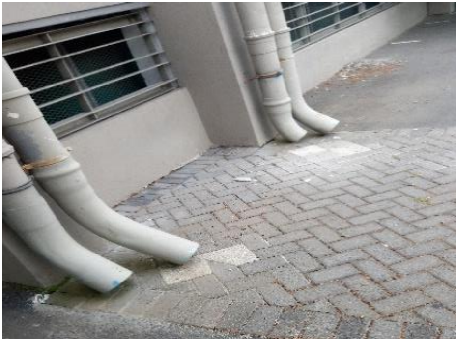
Figure 4-7: Roof downpipes draining onto the PICP
