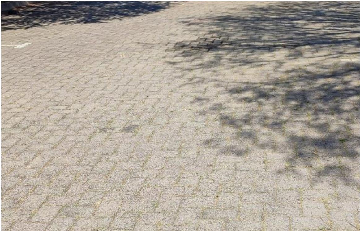
Figure 6-5: PICP surfaces clogged by leaves or pollen from overhanging trees
