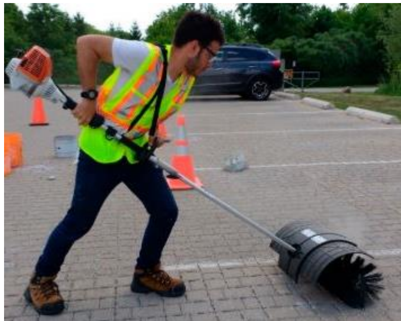
Figure 2-32: Application of a power brush (Sehgal et al. , 2018)
