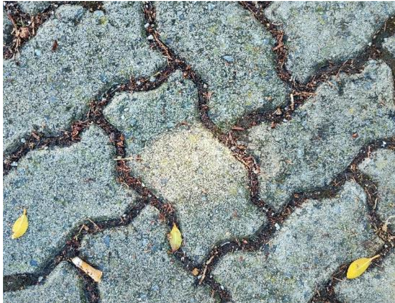
Figure 4-64: Typical Area 2 sediment and organic filled joints
