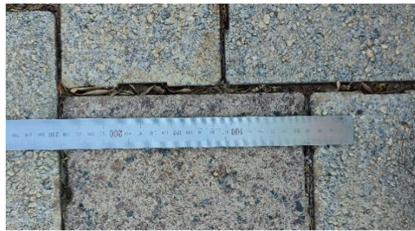
(b) Organic matter filled joints
