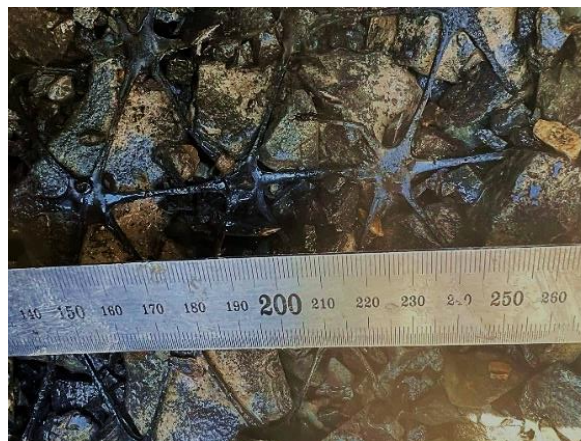
Figure 4-70: Geogrid installation
