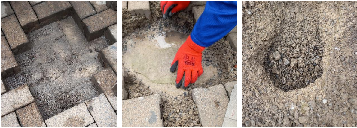
(a) High sediment content (b) High sediment content (c) High sediment content
