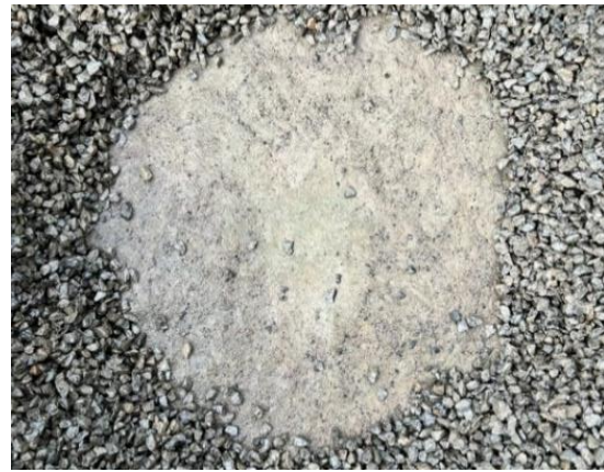
(b) NEB-05 state of the geotextile
