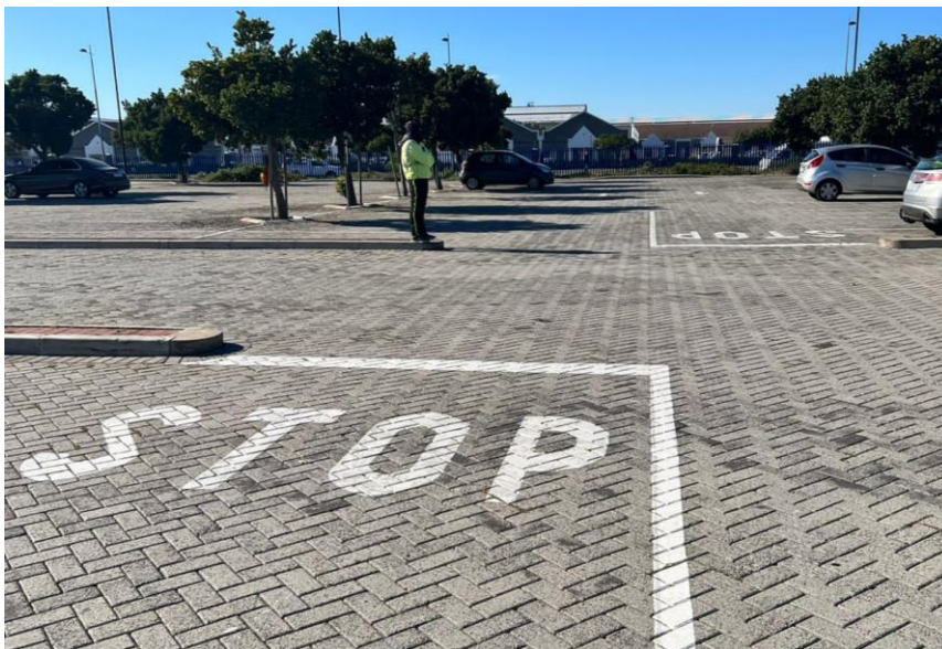
Figure 6-10: Example of well-spaced trees and appropriate edge restraints
