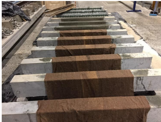
Figure 4.7 Patch repaired RC beams covered with damp Hessian cloth
