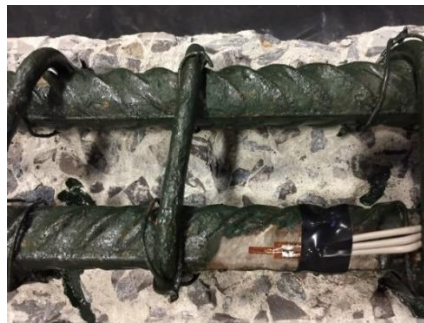
Figure 4.10 Strain gauge installation on tension steel reinforcement
