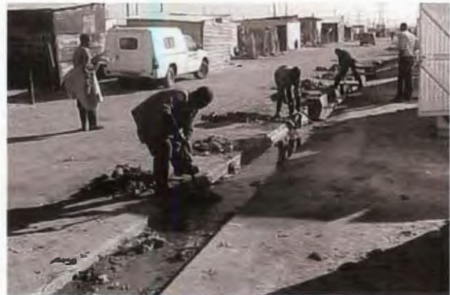
Figure 56 : Stormwater infrastructure in the informal settlement (Bouchard et al., 2007)
