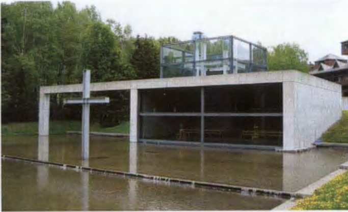
Figure 43: Church on Water (silhvearquitekonica, 2010)
