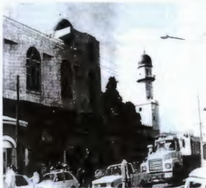
Figure 18: The Grand Anwar mosque with shops along street's side(Hassen,M, 1999)
