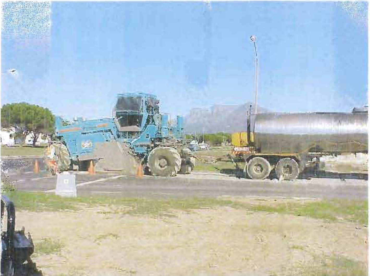
Plate 1 : CTR machine on site
