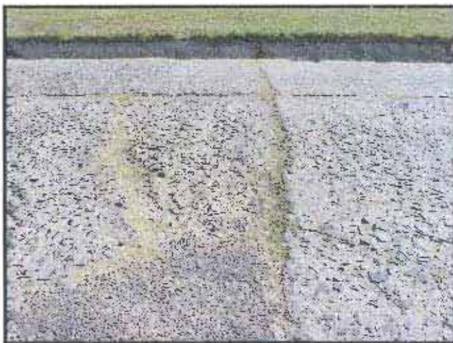
Joint disintegration and raveling resulting in exposed aggregate PLATE 4
