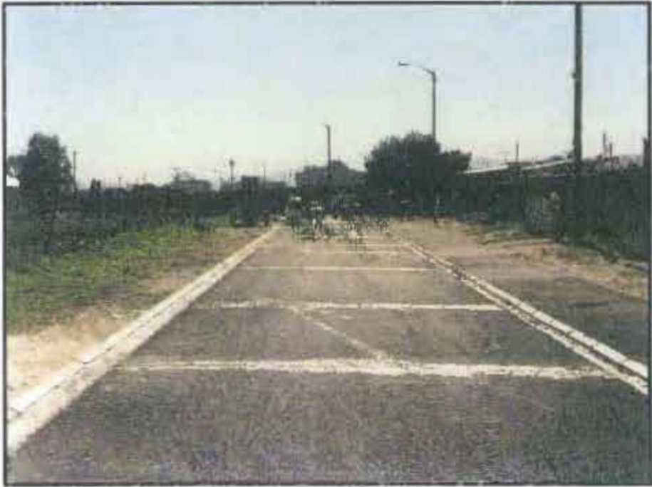
Saw cut joints. PLATE 15
