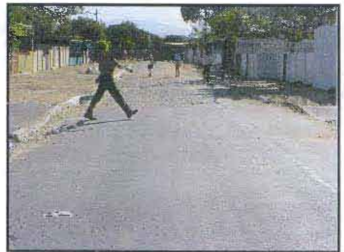
Rubber bitumen asphalt overlay. PLATE 13
